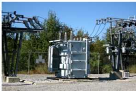
8000 lbs, 60 Hz Distribution Transformer
