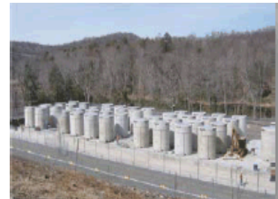
Connecticut Yankee: Nac-MPC MPC canisters
