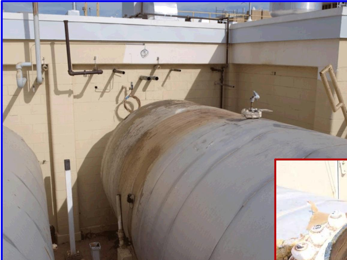
Main pressure lines were cut away as the tank junction.
