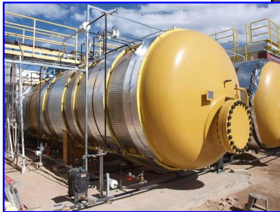
Insulation designed with access panels for the steam jackets.
