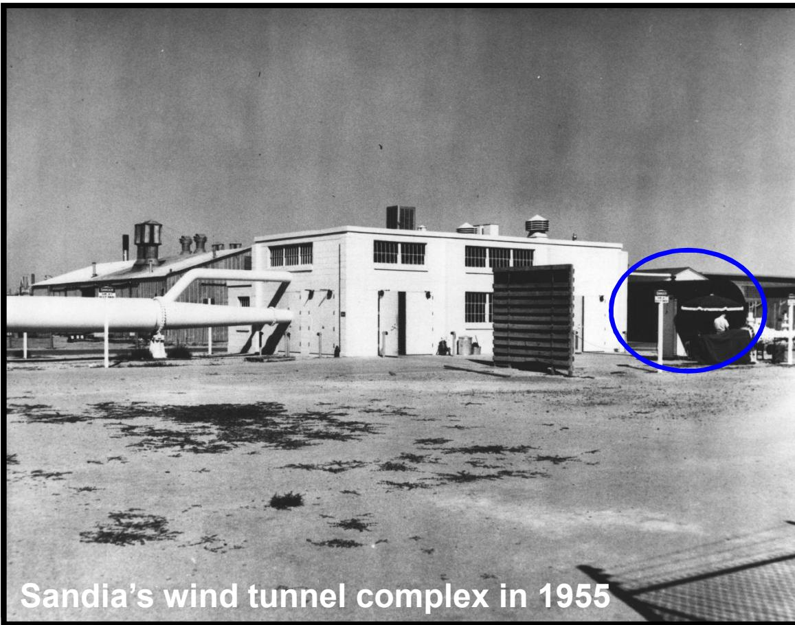
**Initially driven by a single tank of 2600 ft<sup>3</sup> volume, pressurized to 300 psig (74 m<sup>3</sup>, 2 MPa).**
