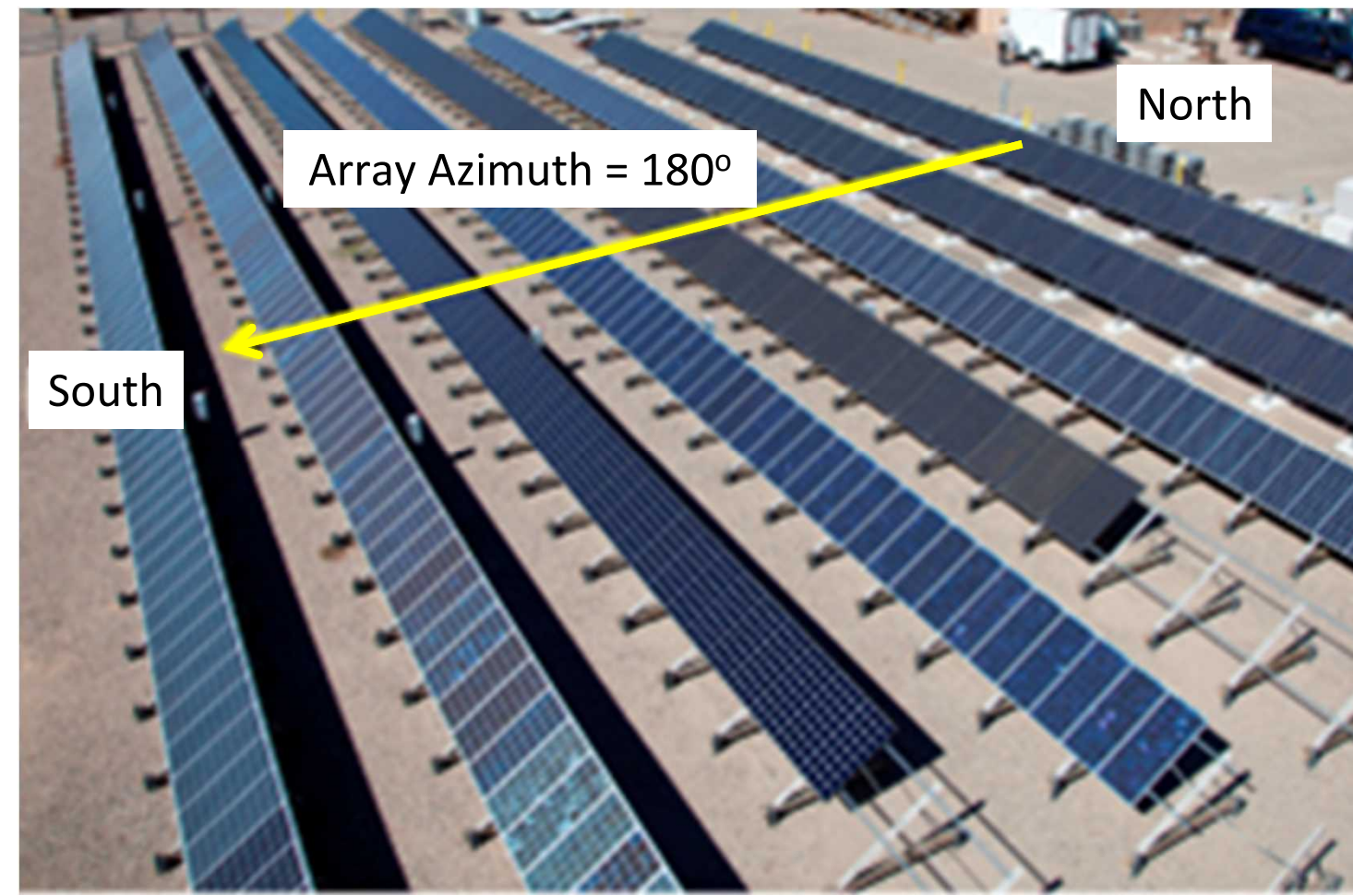
Fixed tilt modules face south at inclination equal to the sites latitude to minimize AOI at solar noon. POA irradiance must be adjusted for AOI and reflection loss.
