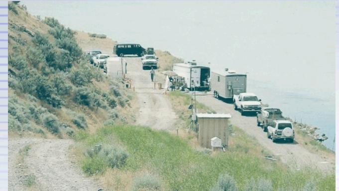
Injection of apatite forming solution at Hanford 100N site for immobilization of Sr-90. June, 2006.
