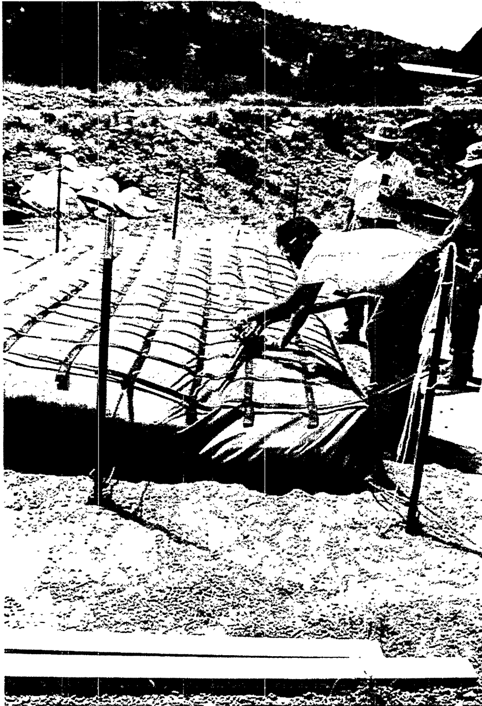
Figure 2. Filling RPF Pontoon Envelopes
