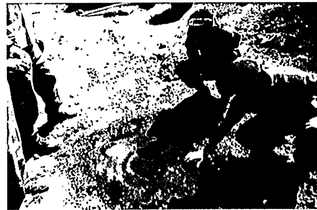
Application of Self-Leveling Polyurethane to Filled "Crater"
