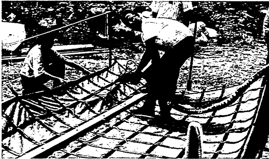
Figure 37. Filling RPF pontoons
