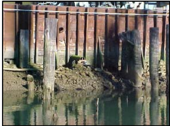
(b) 8-in. and 5.5-in pipes through retaining wall (Y-trap is attached to 8-in. pipe, center of photo)
