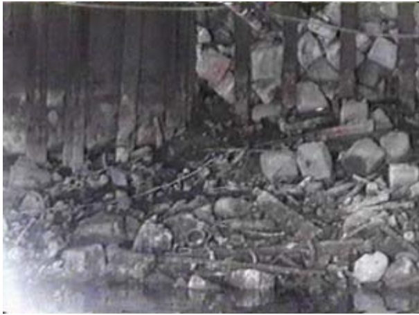
(c) Transition from solid wall to vertical bars holding blocks (~1 ft cubes) of fill material, Transect +26.5
