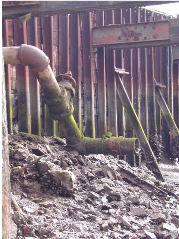
Photo 7 - 'L'-shaped pipe with gate valve. 2/6/02.
