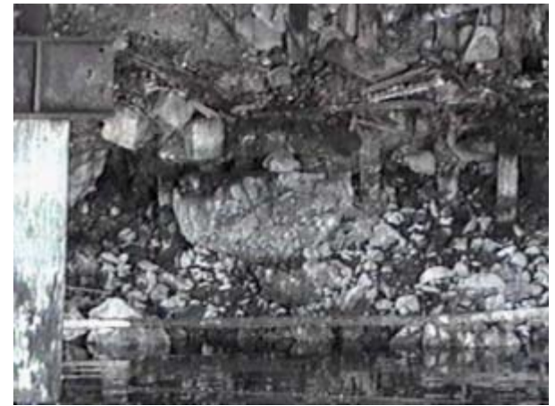
(d) Discontinuity in retaining wall, visible remnants of vertical supports and fill, about Transect +29.5
