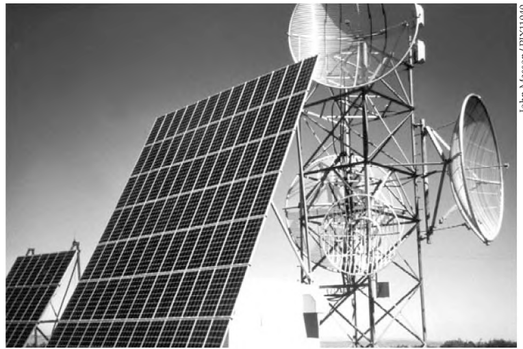
Photovoltaics provides high-reliability power for a communications tower in Dinosaur National Monument.
