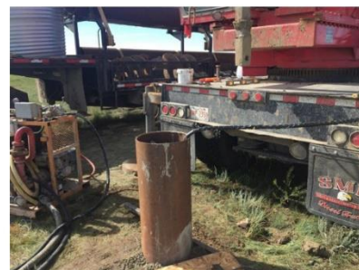
Casing lifted ~3 ft. during cementing
