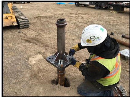
Installing Mounting Plate Drive Tool
