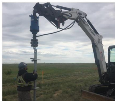
Connecting Skid Steer to first pile
