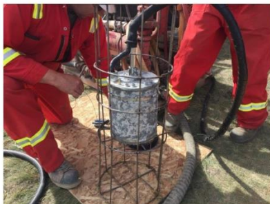
Rebar cage around MicroVib™ unit
