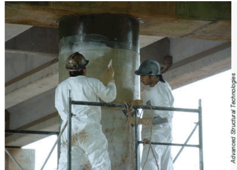
Workers applying GFRP wrap to concrete column (Department of Transportation)
