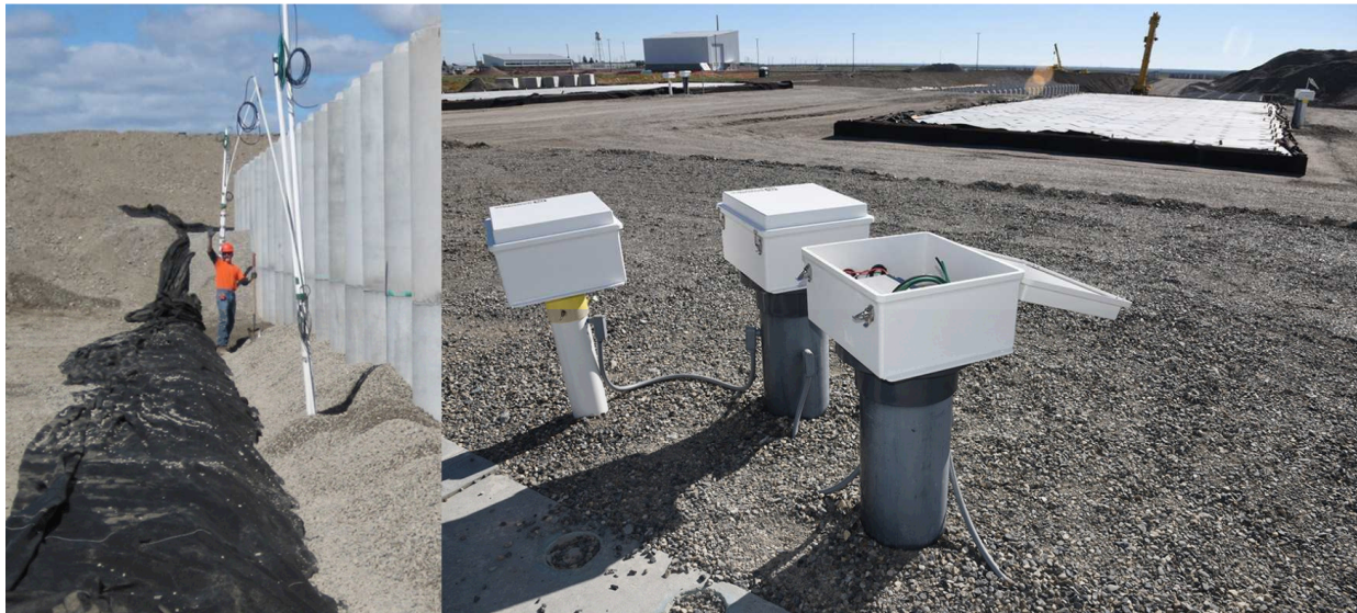
Fig. 6. Monitoring wells (right) and instrument installation during vault construction (left).
