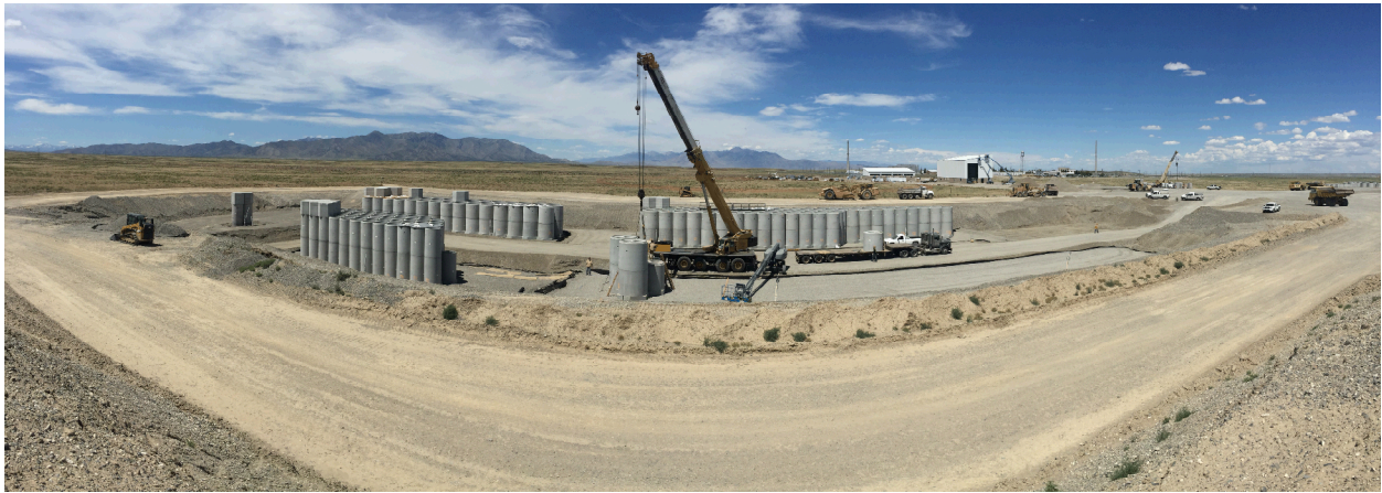
Fig. 3. Vault yard construction showing four all vault arrays.
