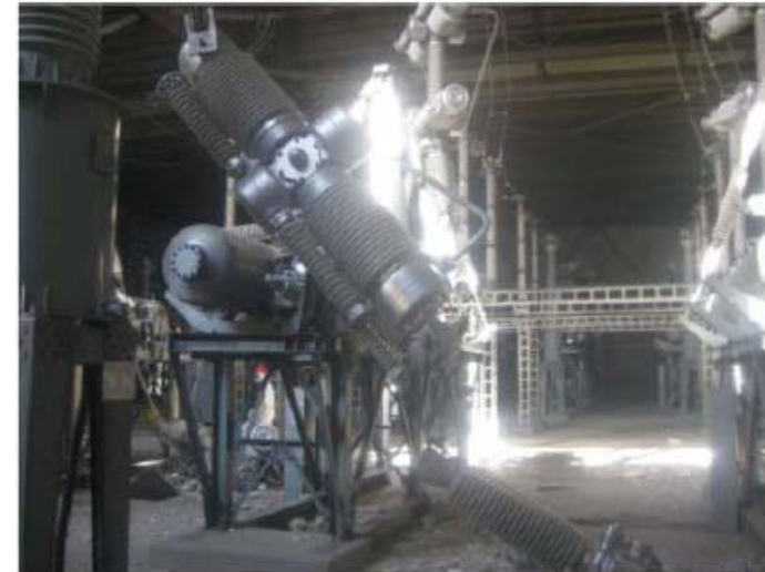
Circuit Breaker damaged
