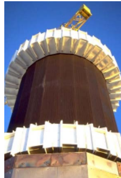
Solar Two Tubular Molten Salt Receiver
