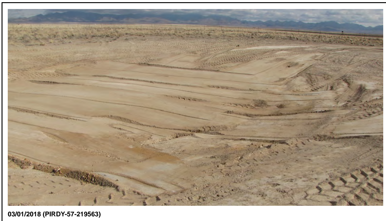
Figure 2-7 SG5, Zone 6 Post-Excavation Facing East
