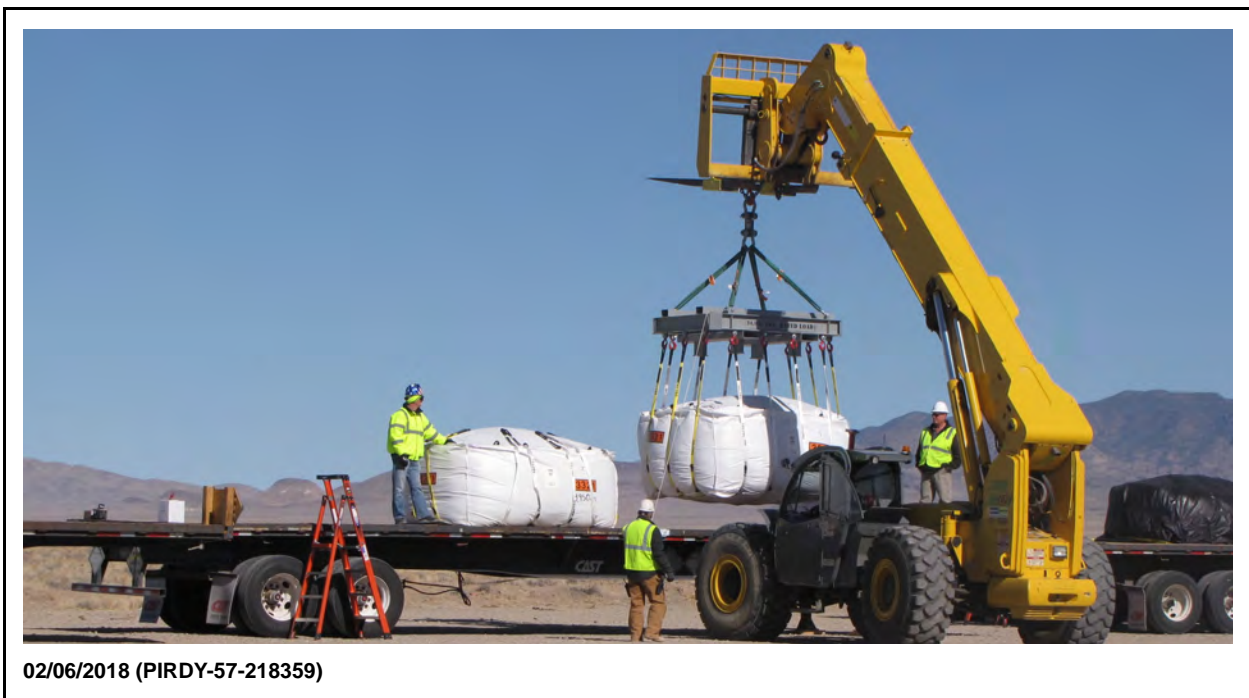
Figure I.1-22 Loading Bags on Flatbed Trailer for Transport to Area 5 RWMC for Disposal Facing Northwest
