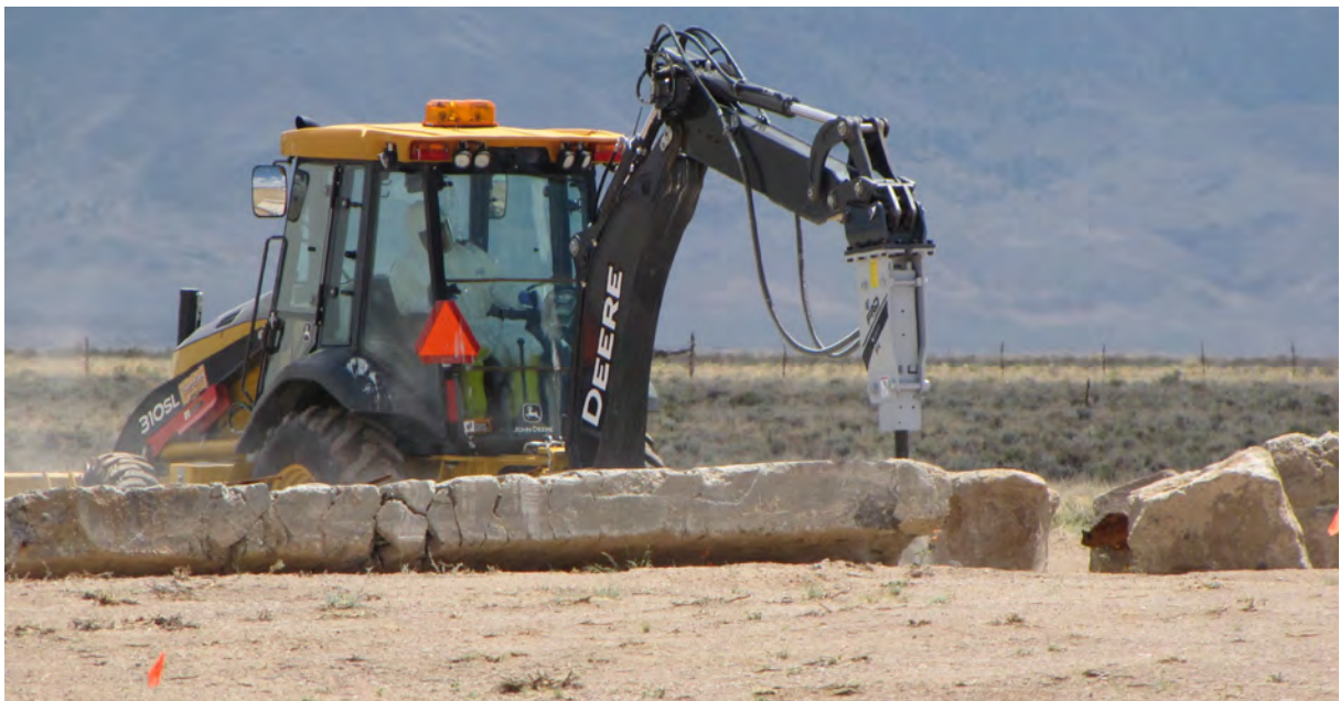
Figure I.1-15 Debris Size Reduction Using Hydraulic Hammer Facing Northeast
