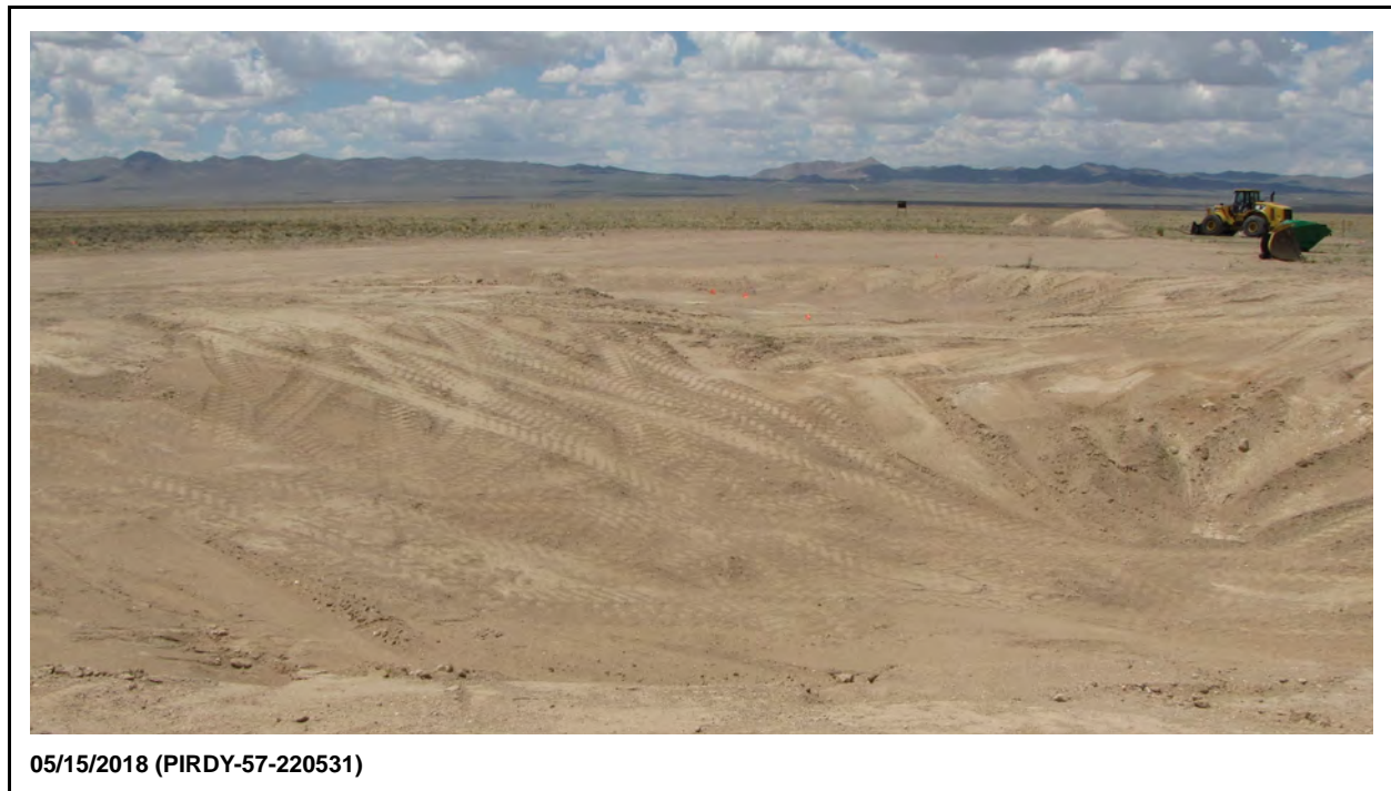
Figure 2-6 SG5, Zone 4 Post-Excavation Facing East
