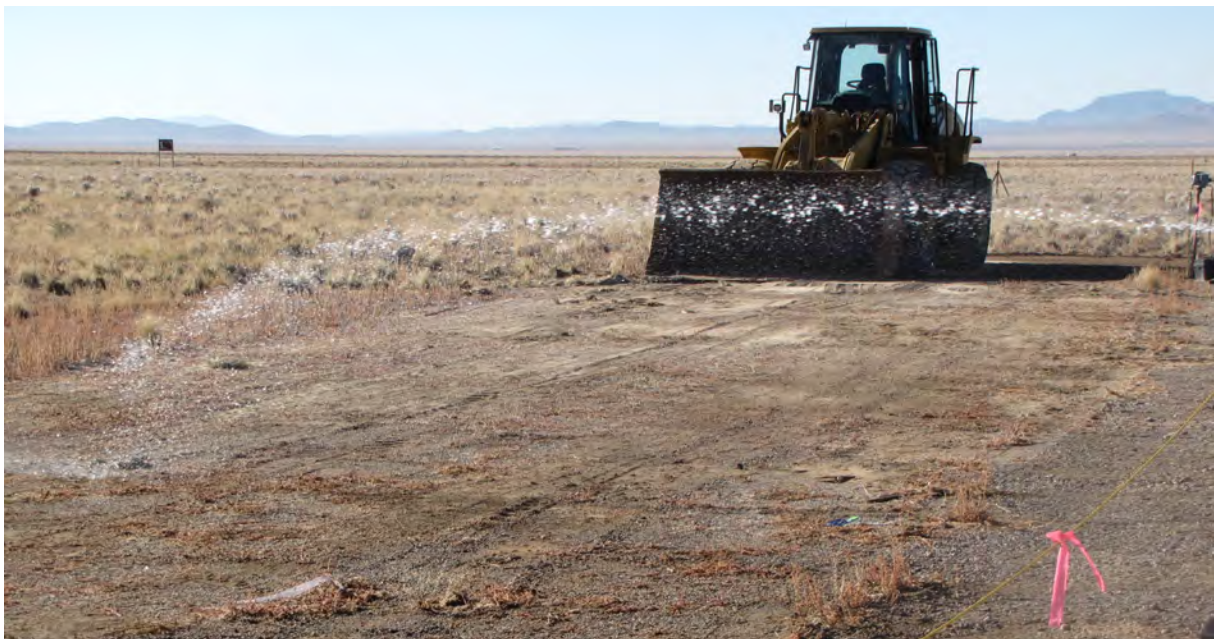
Figure I.1-6 Site Setup Pad Grading and Dust Suppression Facing Southeast
