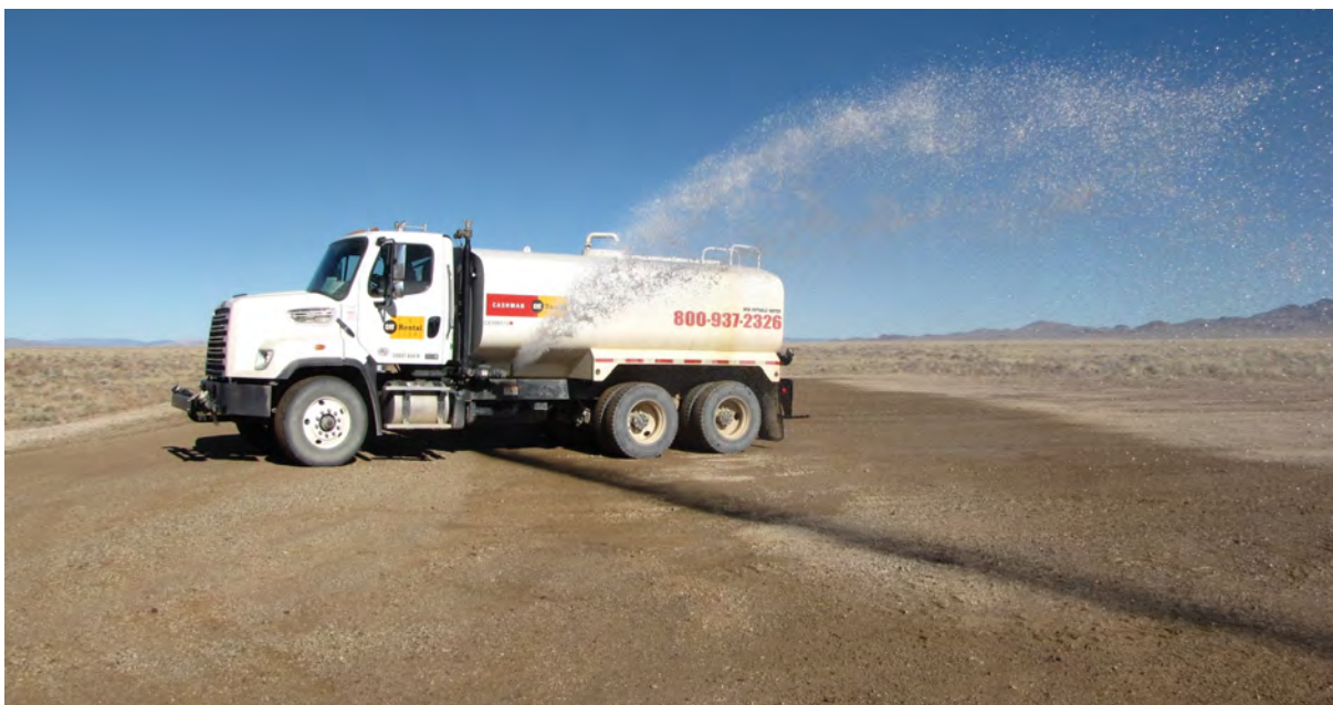
Figure I.1-5 Mock-up Dust Suppression Facing North
