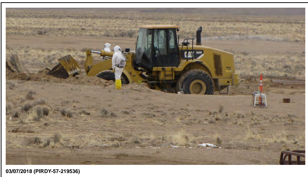
Figure I.1-11 Excavation Activities Facing Southeast
