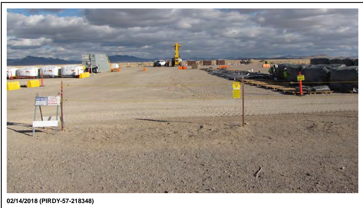
Figure I.1-8 Overview of Site Layout Facing Southeast
