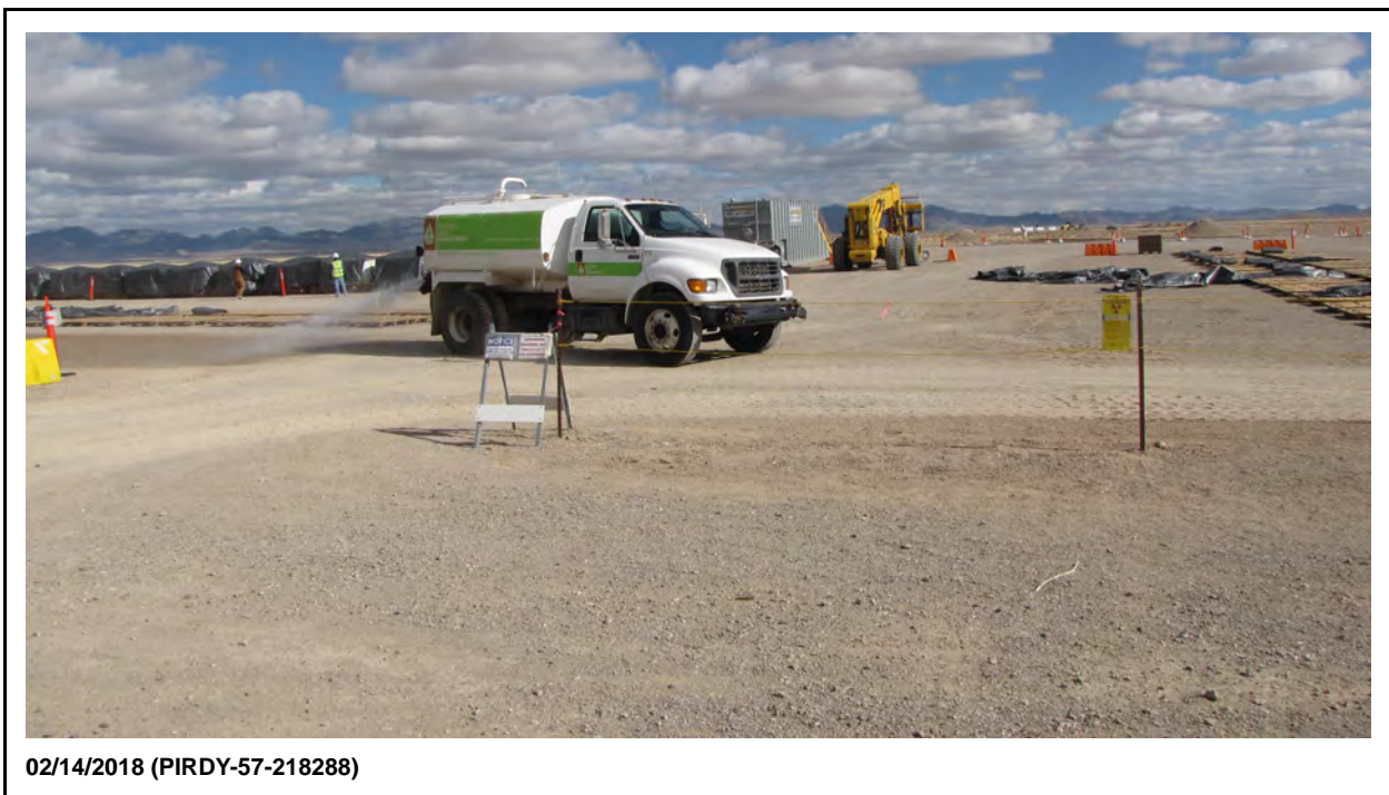
Figure I.1-9 Dust-Suppression Activities in Site Support Area Facing Southeast
