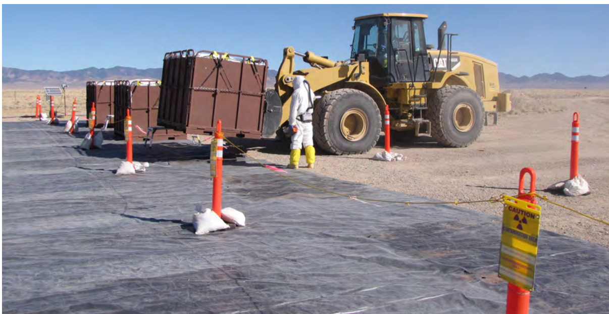
Figure I.1-19 Forklift Transferring Frame and Bag to Radiological Controlled Boundary Facing North
