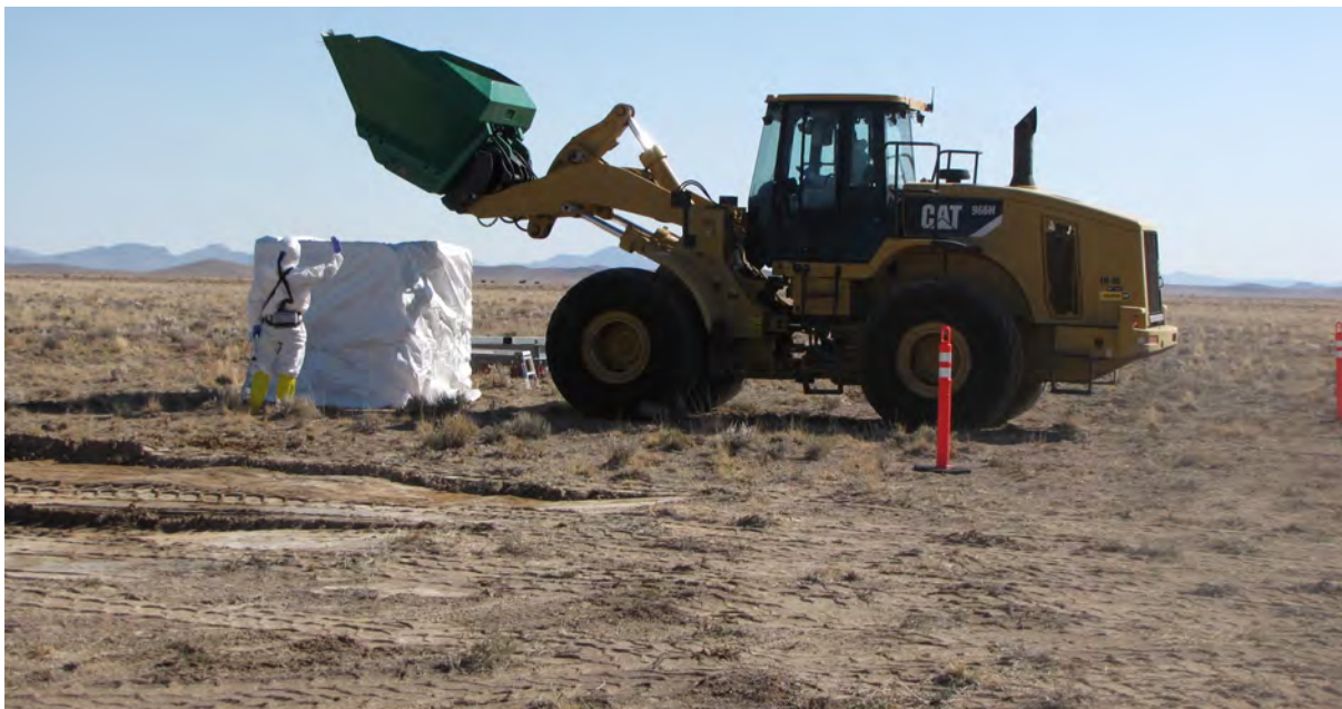
Figure I.1-18 Filling Bags Using Bag-Filling Bucket Facing Northeast
