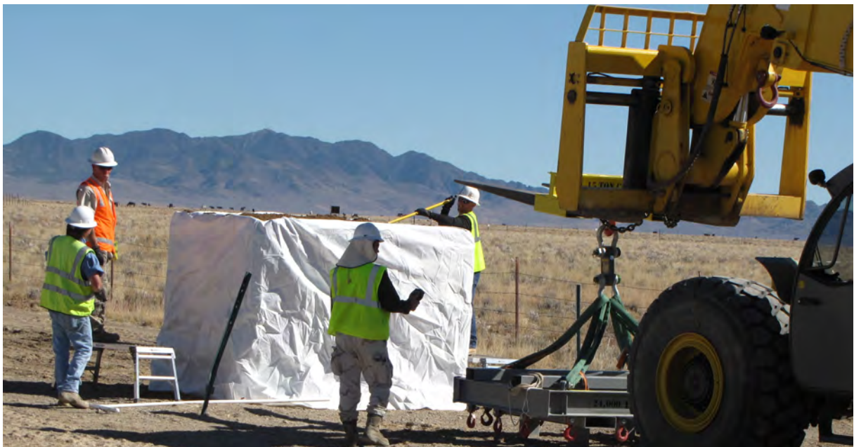
Figure I.1-3 Mock-up of Loading Bags with Clean Soil Facing North
