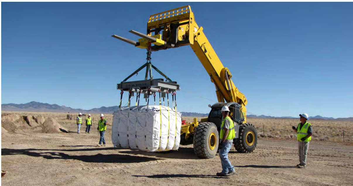
Figure I.1-4 Mock-up Moving Bags Suspended from Lifting Frame Facing North
