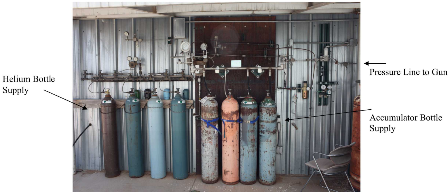
Figure 4. Current Gas Plumbing System
