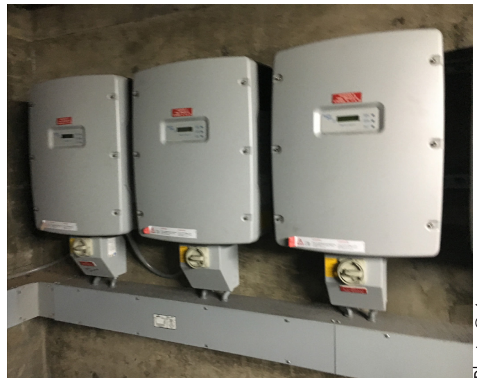
Figure 51: PV inverters
