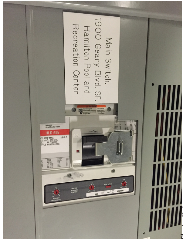
Figure 37: HRC new main electrical circuit breaker
