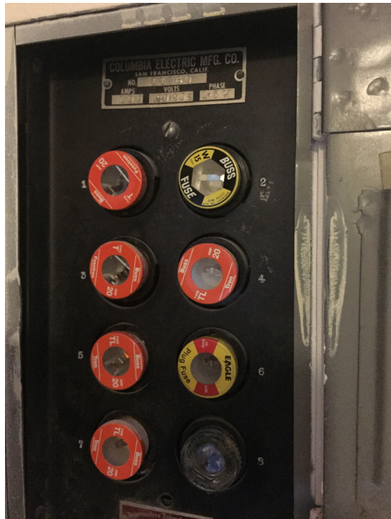
Figure 26: Distribution panel to basement classroom — fuse type panel; difficult to isolate individual circuits easily
