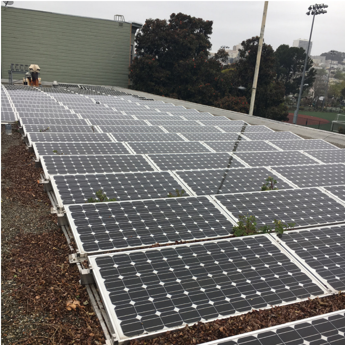
Figure 48: Existing 30 kW PV array
