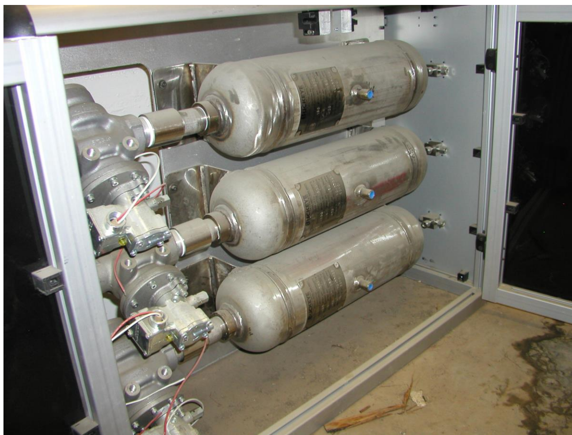
Figure 3: Inside of the accumulator cabinet. By moving critical parts out from under the bridge, maintenance is much more easily managed.
