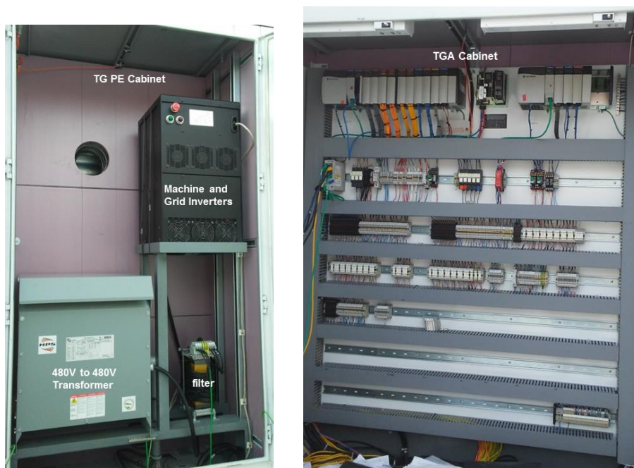
Figure 35 TG PE and TGA cabinets in GM package
