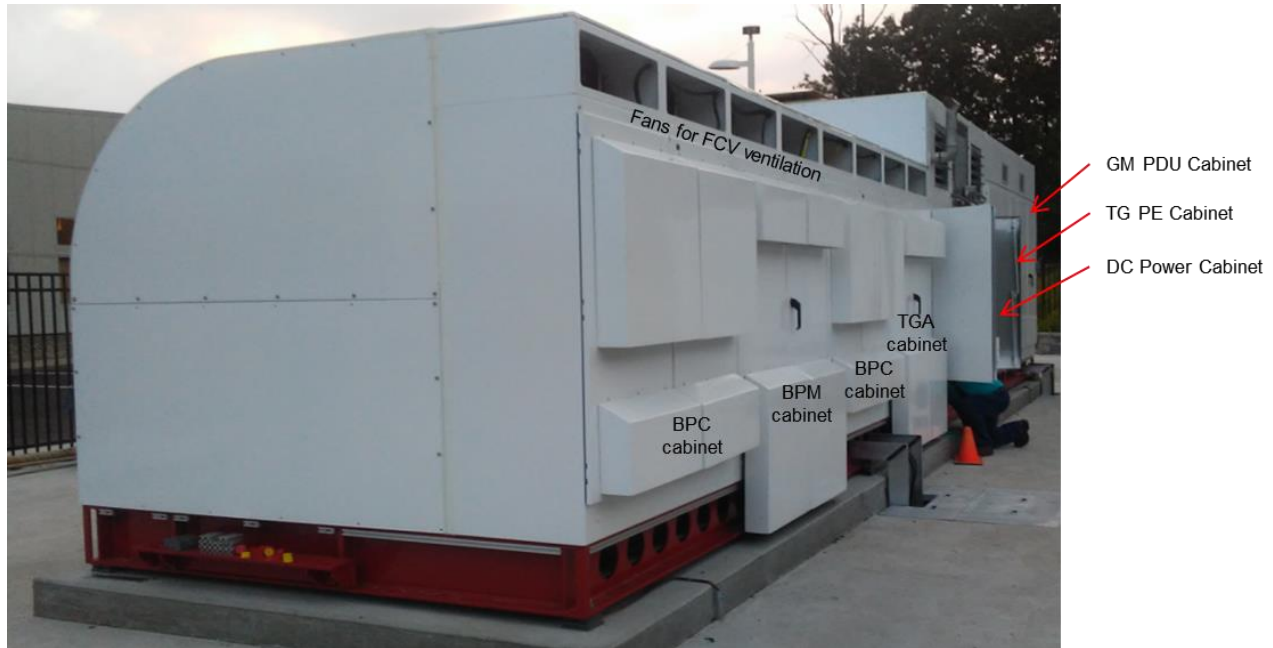
Figure 31 Electrical cabinets in GM package
