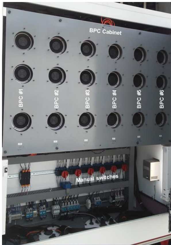
Figure 33 BPC and BPM cabinets in GM package
