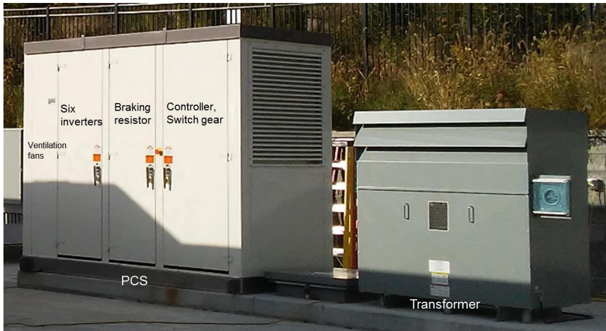
Figure 29 PCS package including transformer
