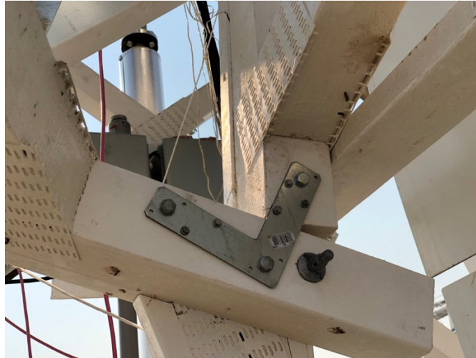
Figure 3-140. Repair of damage due to insufficiency against antiplane shear forces on SRC
