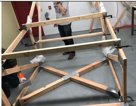
Installation of diagonal members to trusses brackets
