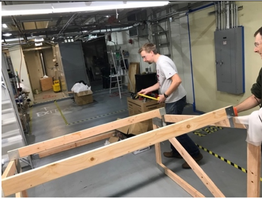
Use of longitudinal rafters to setup truss separation
