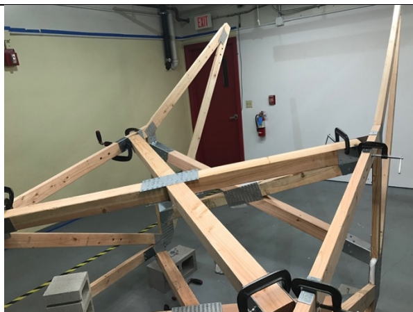
Installation of top diagonal members
