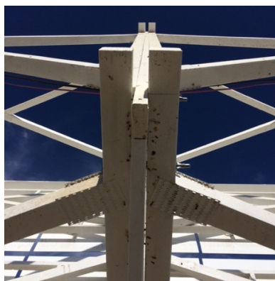
Figure 3-141. Gaps formed within assembly wood to wood joints
