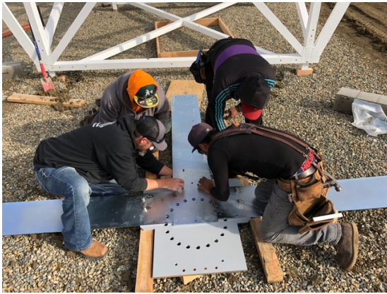
Figure 3-79. End plate assembly
