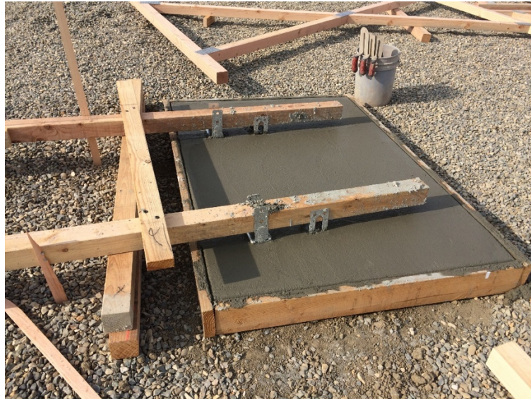
Figure 3-76. Concrete pad for pylons
