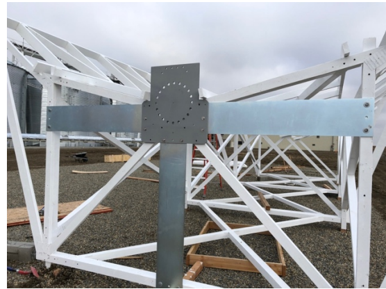
Figure 3-80. End plate on spaceframe
