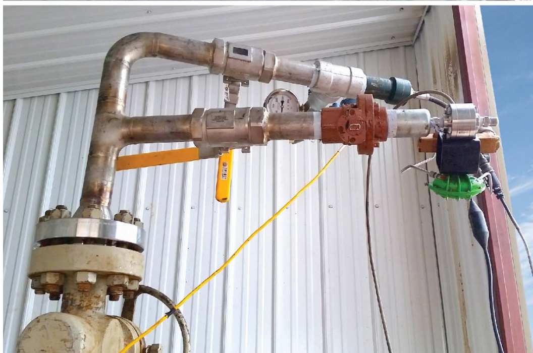
Figure 9. Left: two fabricated flange mounts. Right: a flange mount connected to the top of the CO 2 injection well with source and receiver attached to the horizontal arms.
