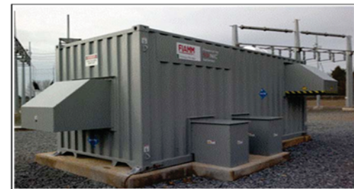
FIAMM 222-kWh System Duke Energy Rankin Substation
