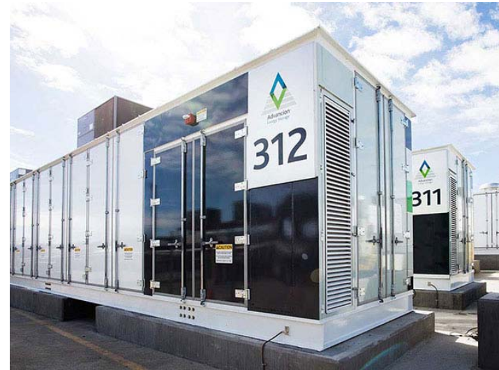
SDG&E 30 MW/120 MWh Li-ion battery energy storage system in Escondido, Calif.
