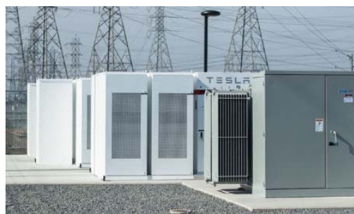
SCE 20MW/80MWh Li-ion Battery Mira Loma, CA
