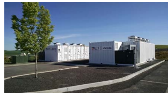
AVISTA 1 MW/3.2 MWh Flow Battery Pullman, WA
