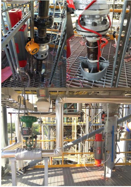
Figure 25. Discharge modifications installed on site. (Top Left) 4" metal seated valve for lock hopper in discharge system; (Top Right) installed heat trace on piping; (Bottom) heat traced, insulated and installed bypass piping and control valve.
