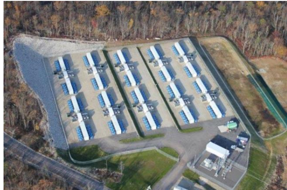
Beacon Power Hazle Township, PA plant. 20 MW, 5MWh. Operational September 2013. Stephentown, NY plant was built first.
