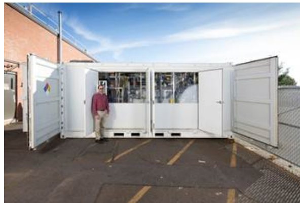
Vionx Vanadium Redox Flow battery, 65kW, 390kWh
