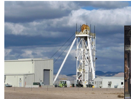
U1a Facility at Nevada National Security Site
