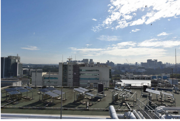
Fig. 1. Test setup for monitoring the long-term performance of PV modules on the rooftop of a building at the NUS campus.
