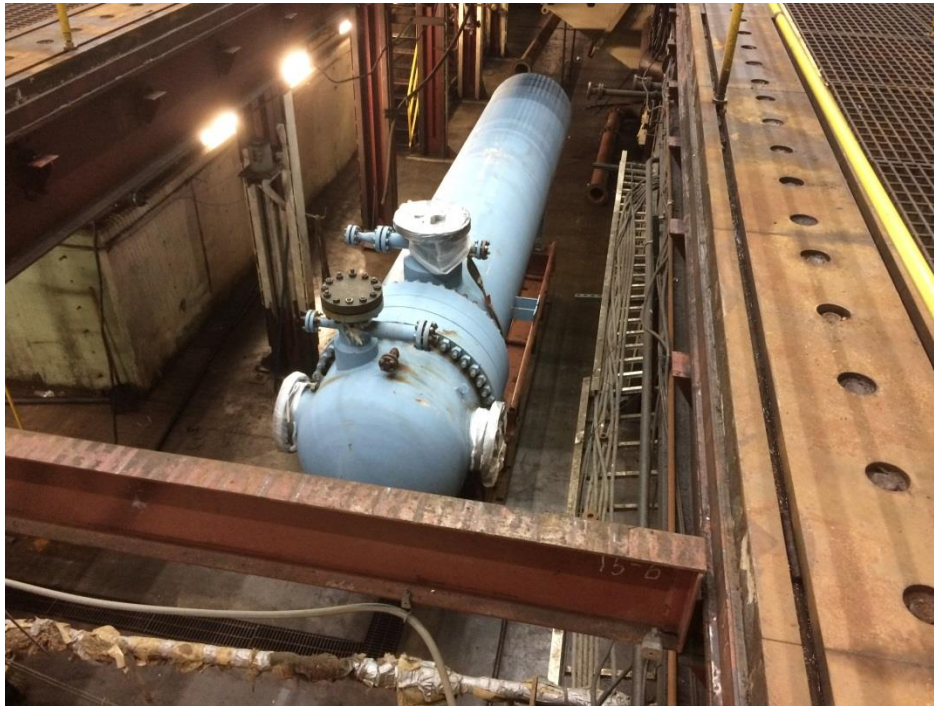
Figure 14 – Flow Loop Cooler
