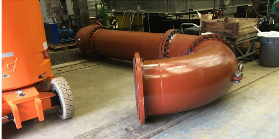
Figure 12 – Suction Piping Assembly
