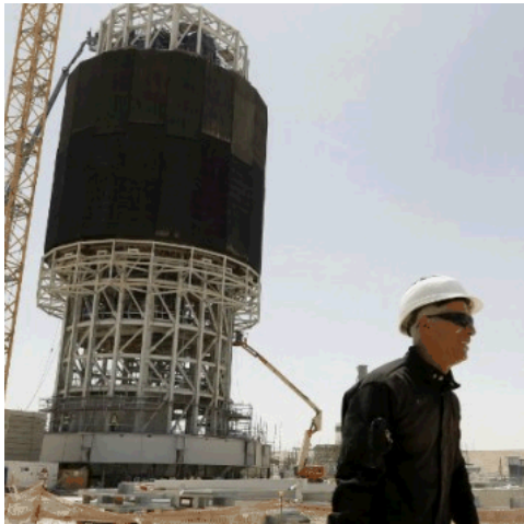
Receiver and heliostat field under construction
