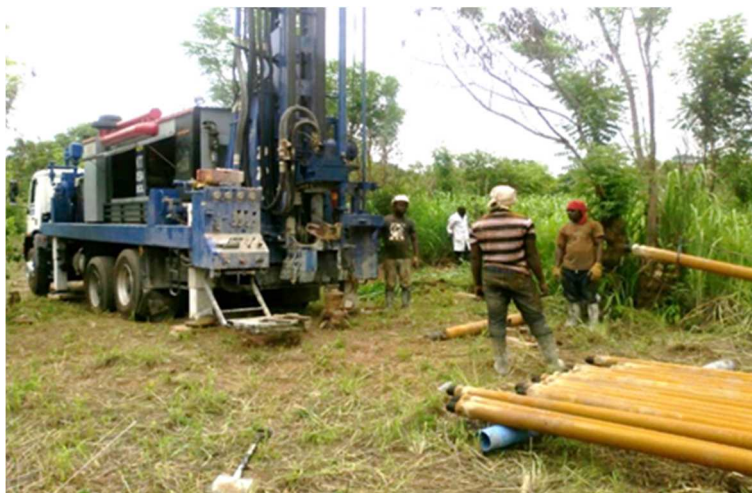
Fig. 10. Drilling One of the Site Characterization Boreholes at the GAEC Site
