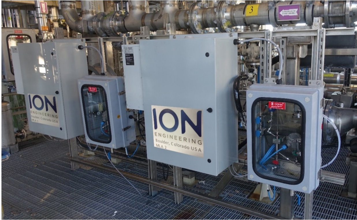
Figure 14 – MLA units installed in weatherproof enclosures at TCM.
