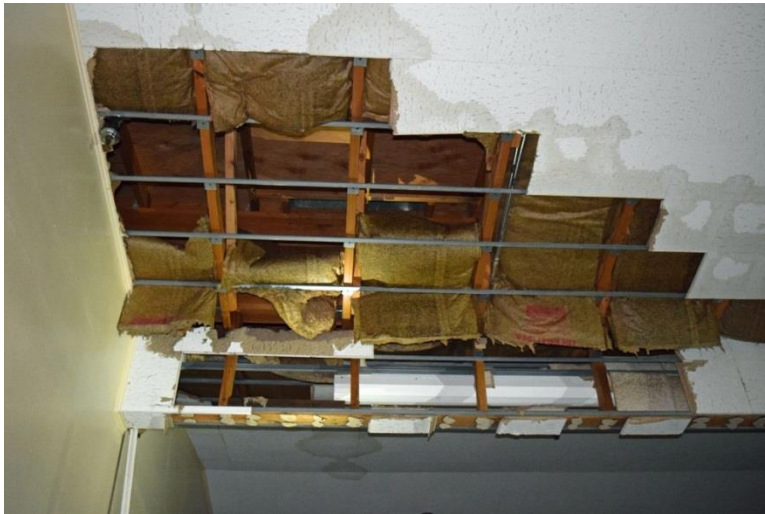
Figure 15. Interior water damage. Top left: Circulation Corridor (112). Top right: laminated bowling lane pushing through the Recreation Room (108A) floor. Bottom: ceiling above Bowling Lanes (102) (DRI 2016).
