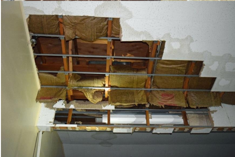
Interior water damage. Top left: Circulation Corridor (112). Top right: laminated bowling lane pushing through the Recreation Room (108A) floor. Bottom: ceiling above Bowling Lanes (102) (DRI 2016).
