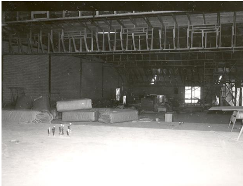
Figure 16. Typical bent assembly. This photo of the northeast portion of the building during construction shows a bent assembly. The steel I-beam posts are visible in the wall prior to being covered by mortar pilasters. The principal roof support along the narrow axis is the glue-lam beam visible along the top of the photo. Supplementary framing surrounding the beam provided additional shear resistance along with provision for sound dampening, lighting, and air flow (REECo Photo 1673-6, 1963-1964).
