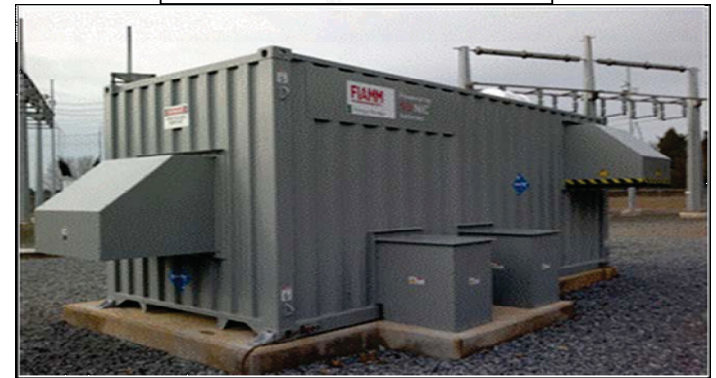
FIAMM 222-kWh System Duke Energy Rankin Substation
