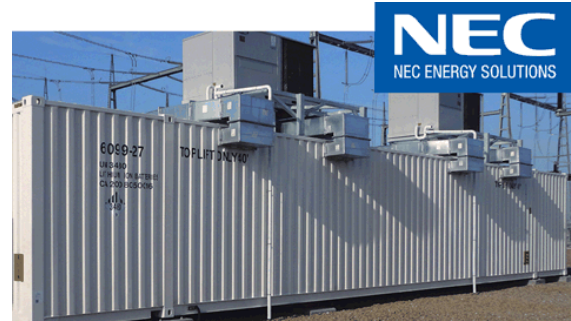
2 MW/3.9 MWh ES System at Sterling Municipal Light Department, Sterling, MA
