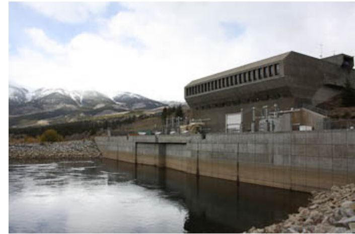
Mt. Elbert Pumped Hydro, 0.2MW, peaking plant, operational 1981.
