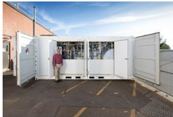
Vionx Vanadium Redox Flow battery, 65kW, 390kWh
