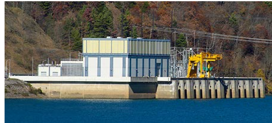
Bath County Pumped Storage (Dominion Resources), 3 GW, operational December 1985
