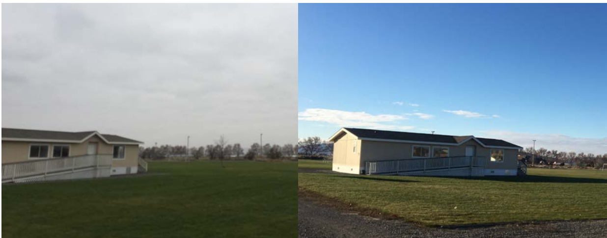
Figure 4.11. Savings Realized with Shades Pulled Down on a Cloudy Day (left photo taken on December 11, 2017, HVAC savings of 5% realized on this day). Negligible or negative average watt-hr/day savings realized on sunny days with few clouds (e.g., negative savings on December day with few clouds, right photo).
