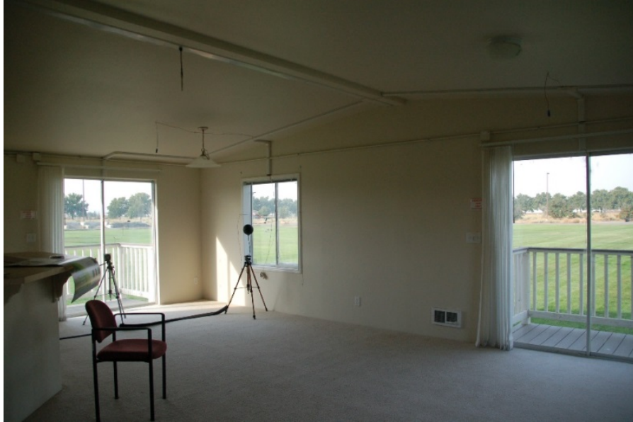
Figure 4.4. Large West- and South-Facing Windows in Common Area Rooms Allow Considerable Heat Gains in when not Fully Covered by Window Shading
