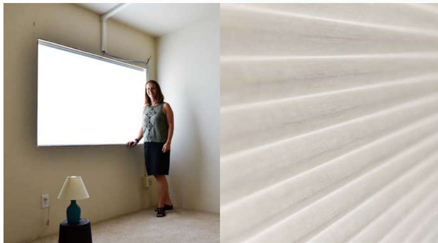
Figure 3.2. Semi-Opaque Double-Cell Shade Pulled Down (left) Allows Filtered Natural Light into North-Side Bedroom. Close-up view of same shade (right).
