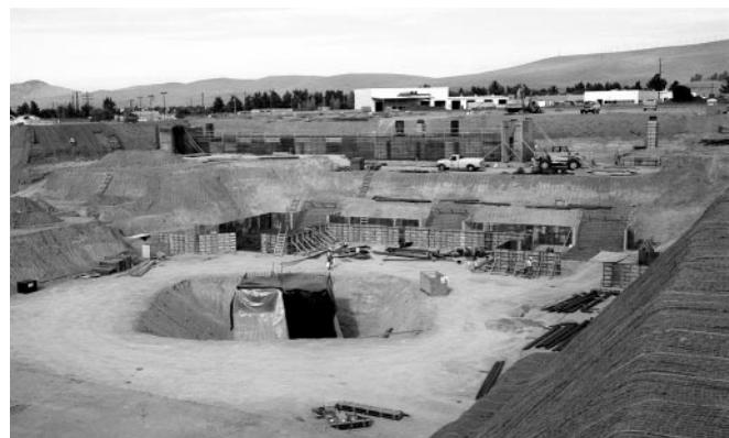
FIGURE 15. Excavation and forms for the NIF target area at year's end. (40-60-1197-2342#1pb01).
