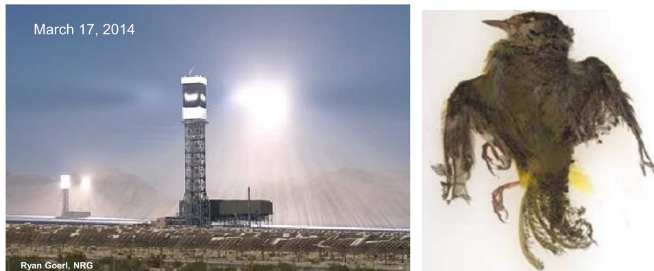
Figure 12. Left: Illuminated standby aim points next to the receiver at Ivanpah using original aim-point strategy before changes were made. Right: MacGillivray Warbler with “Grade 3” solar flux injury found at Ivanpah [19].
