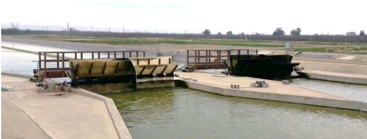
Figure 70: Paddle wheel station. Each raceway is mixed by paddle wheels 2.4-m in diameter and 6.1-m long.
