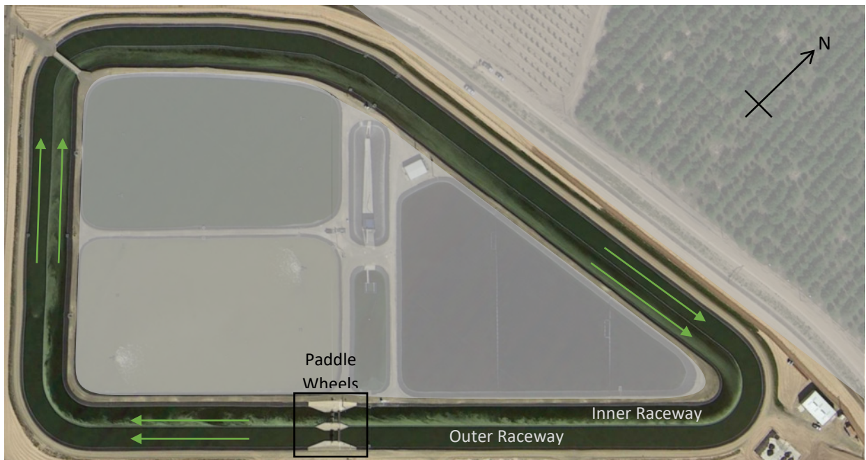
Figure 69: Aerial View of the Delhi, Calif. Wastewater Treatment Facility. The facility has two algae raceway ponds surrounding it, an inner and outer.
