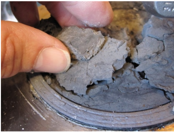
Figure 112: Mineral Deposits on Filter
