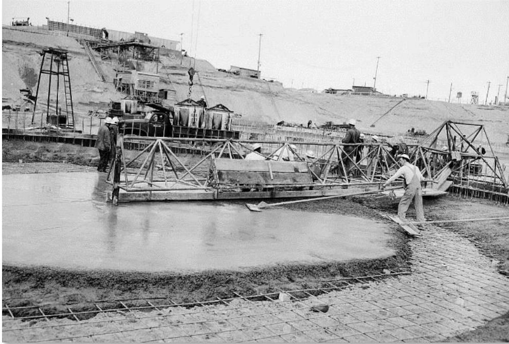
Figure 4-9: Pouring of Concrete in Base Slab Showing Wall Dowels Around the Perimeter (RPP-PLAN-61510)
