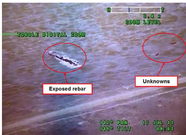
Figure 4-38: Exposed Rebar in Tank S-109 (RPP-RPT-55951)
