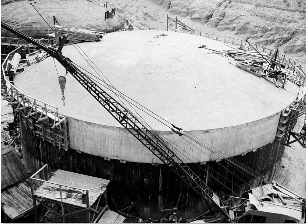
Figure 4-23: Removal of Exterior Forms from Dome Concrete (RPP-PLAN-61510)
