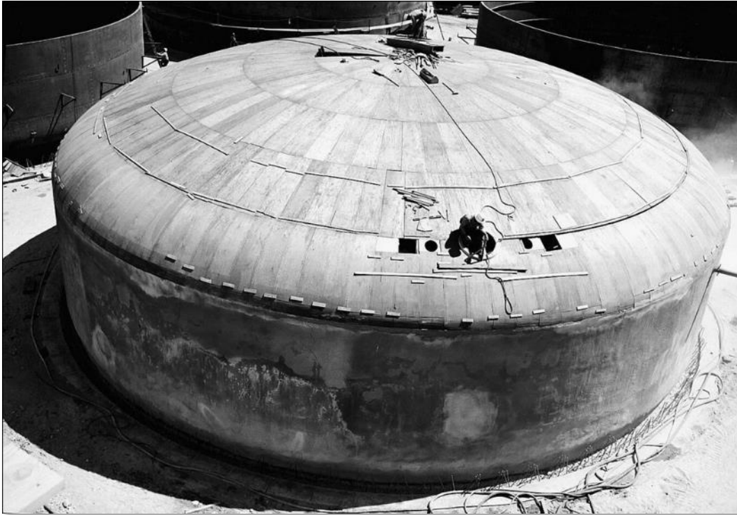
Figure 4-15: View of Liner Coating and Wood Forms for Dome Concrete (RPP-PLAN-61510)
