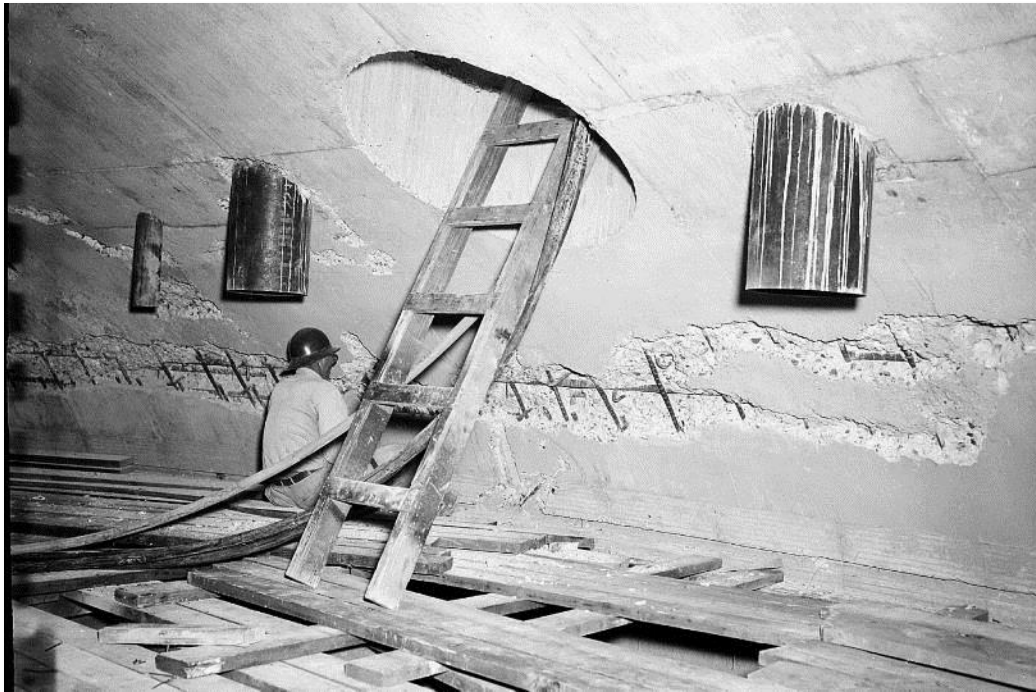
Figure 4-28: Interior of Tank Dome Showing Dome Penetrations and Repair of Construction Flaws (RPP-PLAN-61510)
