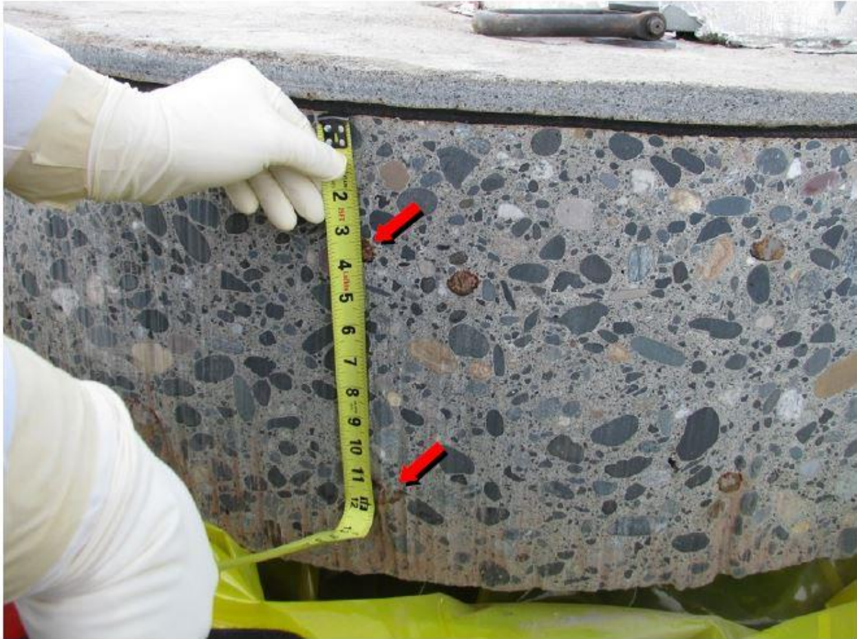
Figure 4-35: Typical View of the Concrete Reinforcing (RPP-RPT-50934)
