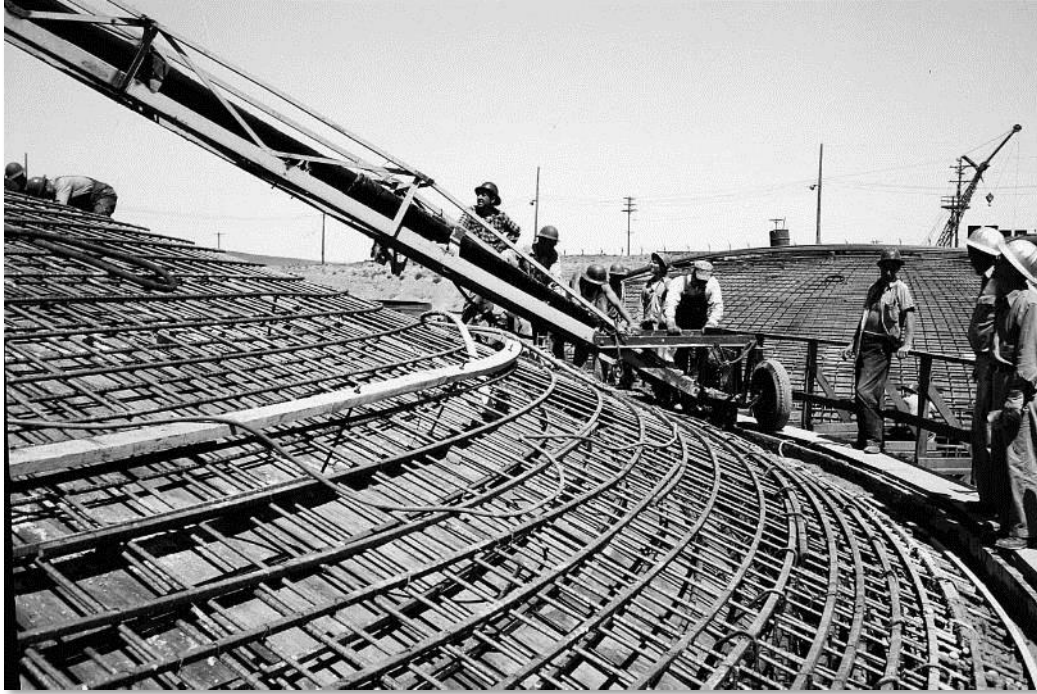
Figure 4-19: View of Dome Reinforcing Steel Showing Square and Deformed Round Bars (RPP-PLAN-61510)
