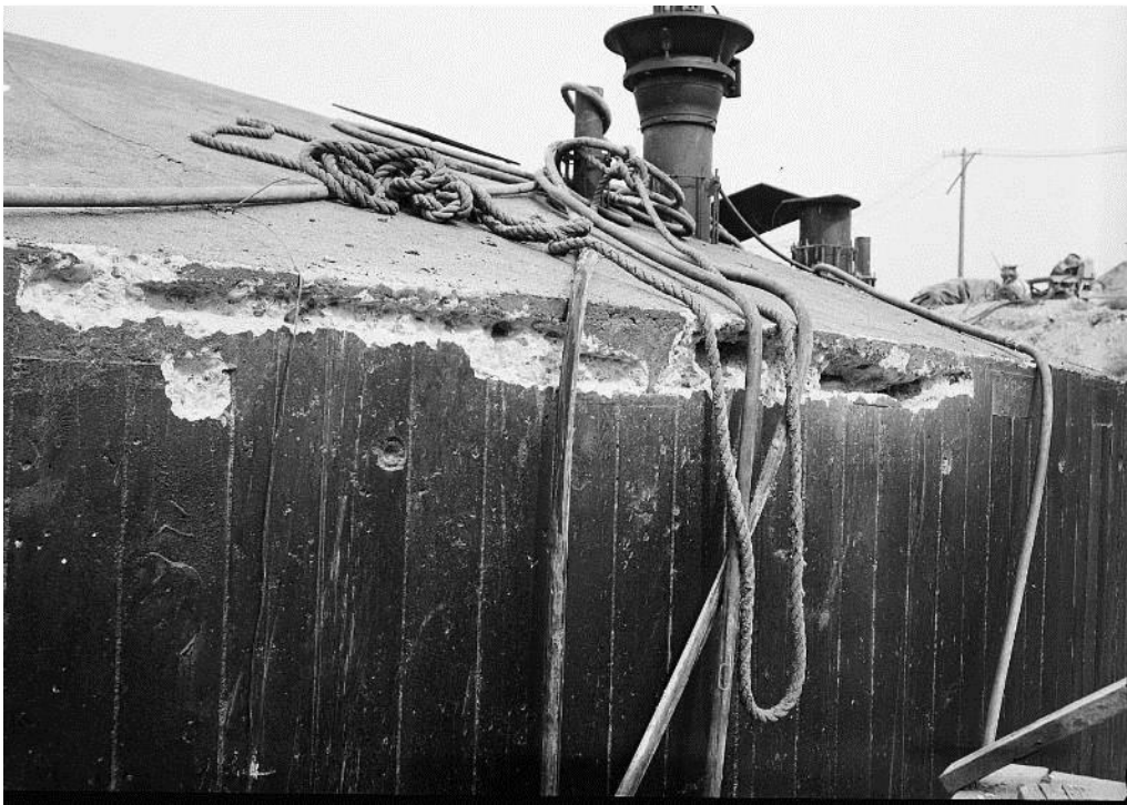
Figure 4-24: Voids in Concrete Created During Construction (RPP-PLAN-61510)
