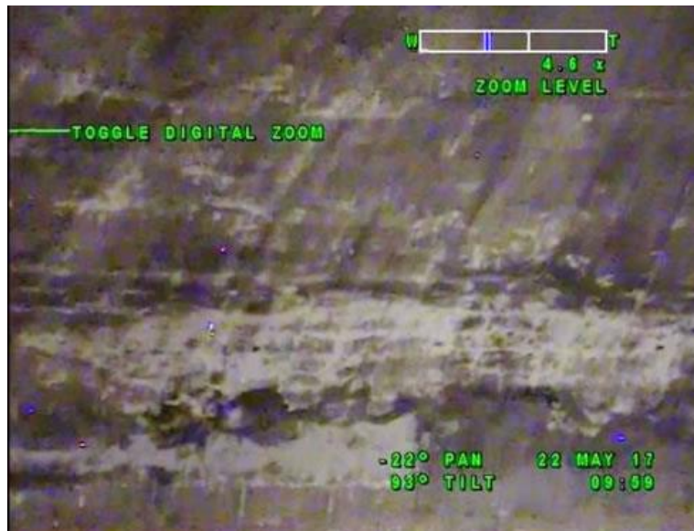
Figure 4-42: Previous Concrete Repair on Tank BX-107 (RPP-RPT-60093)
