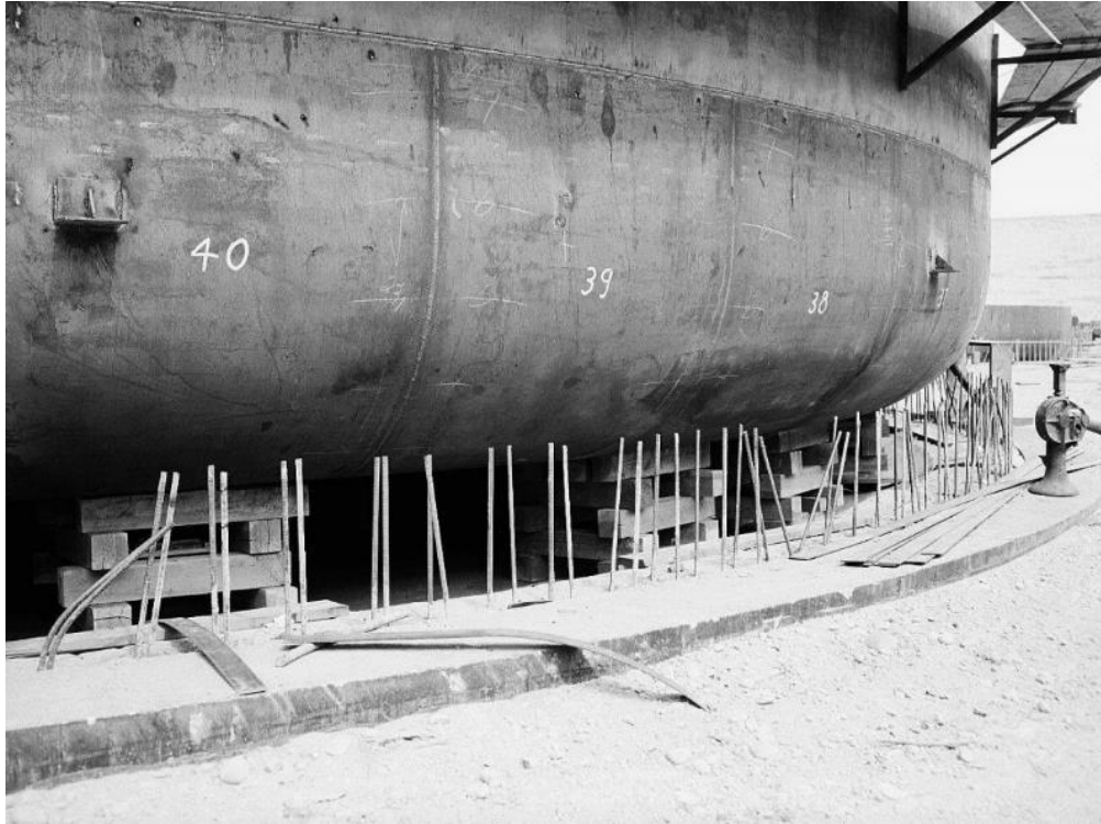
Figure 4-13: Transition from Tank Base to Vertical Wall BX Tank Farm (RPP-PLAN-60765)
