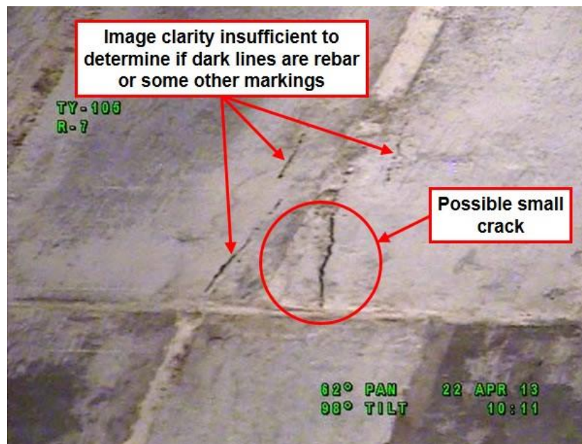
Figure 4-39: Possible Cracks in Tank TY-105 (RPP-RPT-55951)
