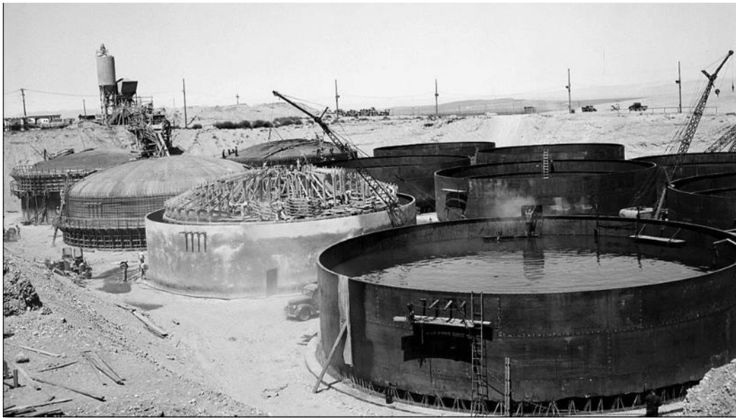
Figure 4-14: Tanks in Various Stages of Construction Showing Hydrostatic Testing of Liner (RPP-PLAN-61510)
