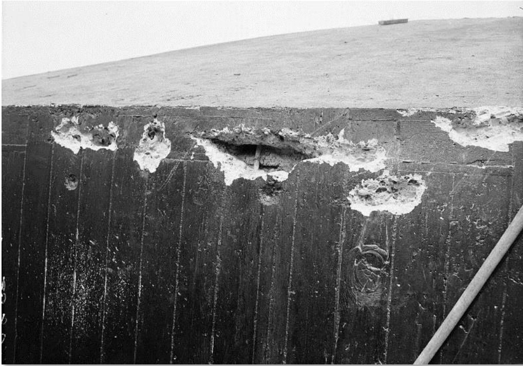
Figure 4-25: Voids in Concrete Created During Construction Showing Reinforcing Steel (RPP-PLAN-61510)
