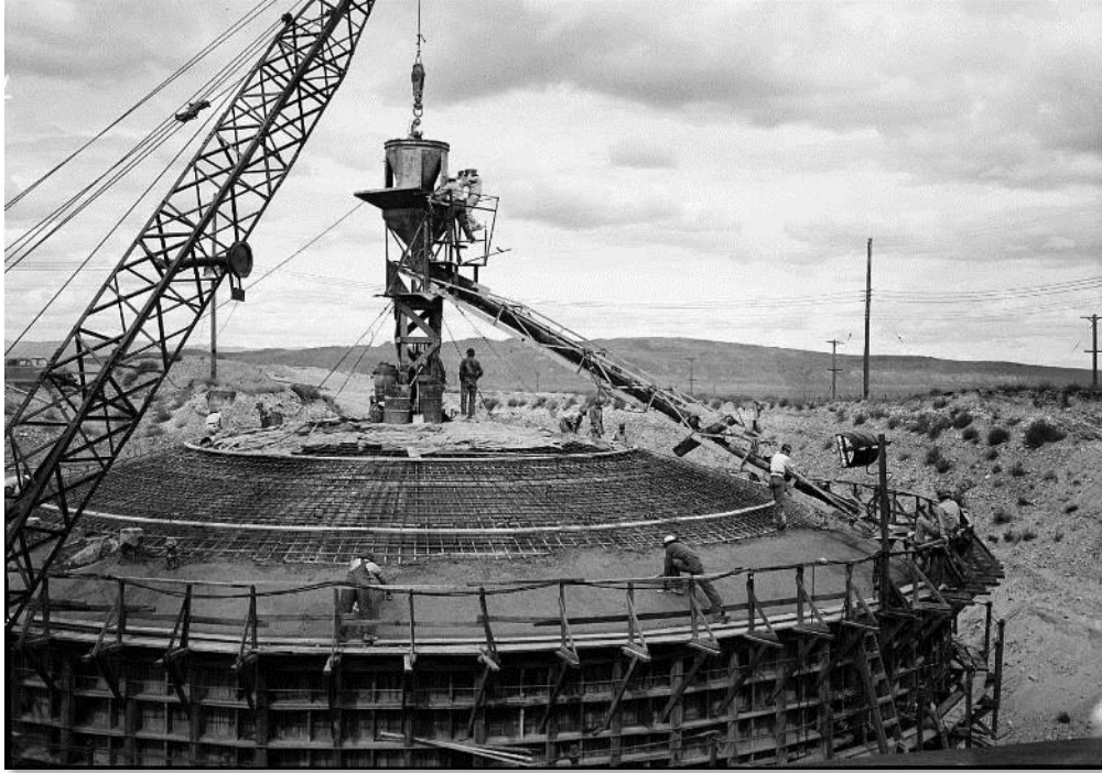
Figure 4-21: Pouring of Dome Concrete (RPP-PLAN-61510)
