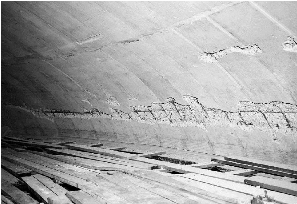
Figure 4-26: Interior of Tank Dome Showing Construction Flaws and Visible Form Lines (RPP-PLAN-61510)
