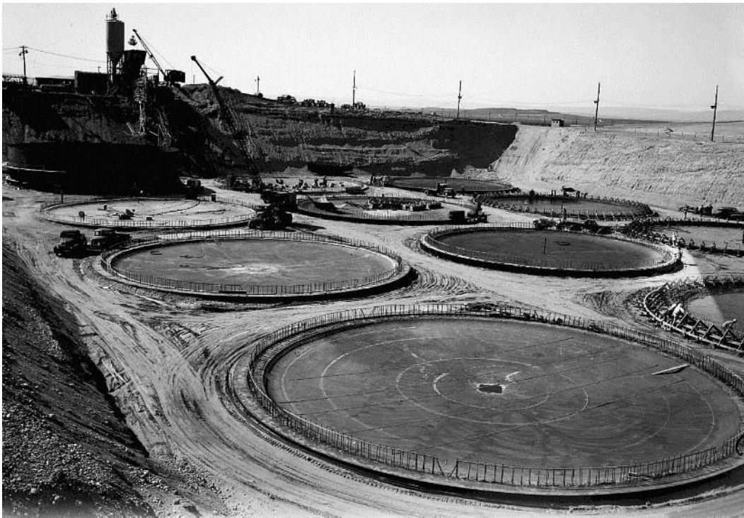
Figure 4-10: Base Slab Construction (RPP-PLAN-61510)
