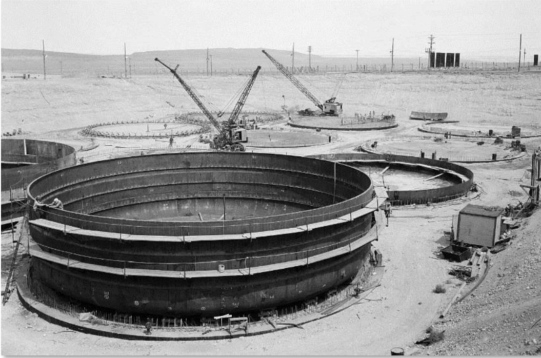
Figure 4-11: Construction of Steel Liners (RPP-PLAN-61510)
