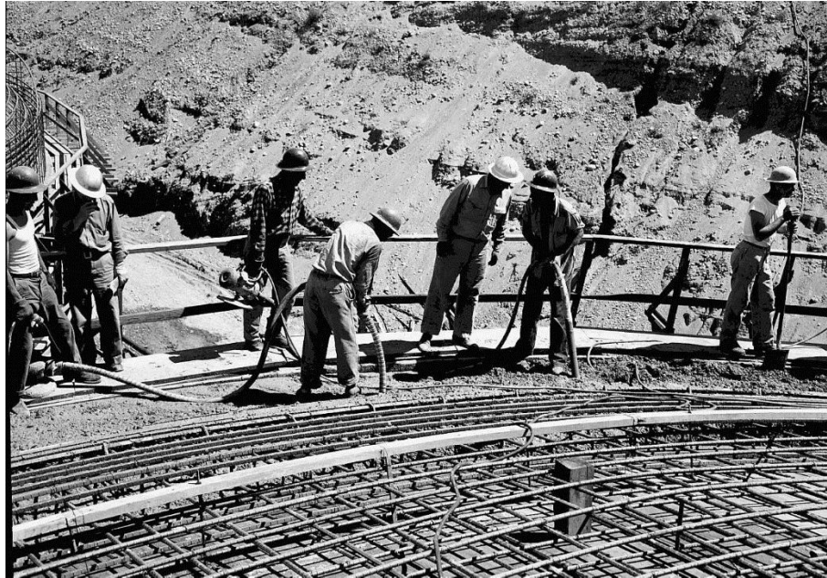
Figure 4-22: Dome Concrete Being Vibrated BX Tank Farm (Photos 1326-Neg [1947] BX Tank Farm Progress)
