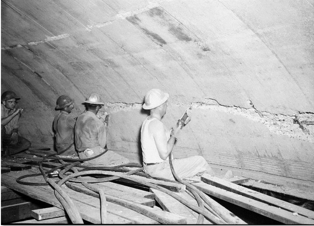
Figure 4-27: Interior of Tank Dome Showing Repair of Construction Flaws (RPP-PLAN-61510)
