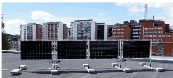
Figure 2: Vertical bifacial array in Turku, Finland.
