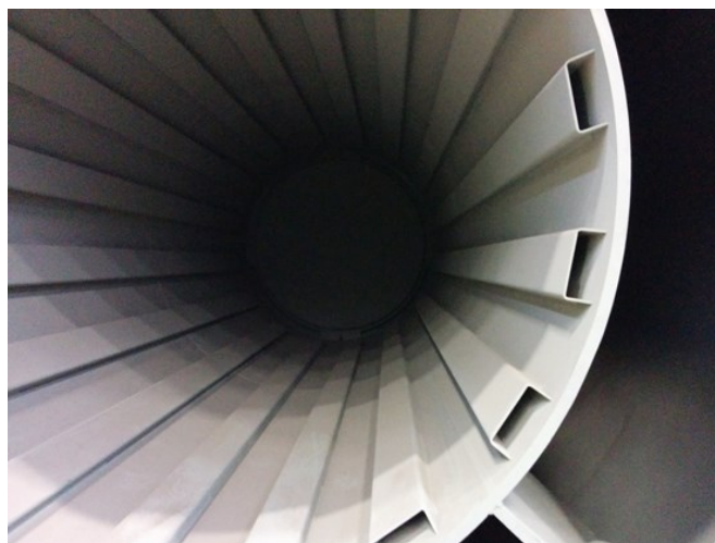
Figure 2.2.2. Carbon steel guide channels on the steel clad interior of the HI-STORM overpack.
