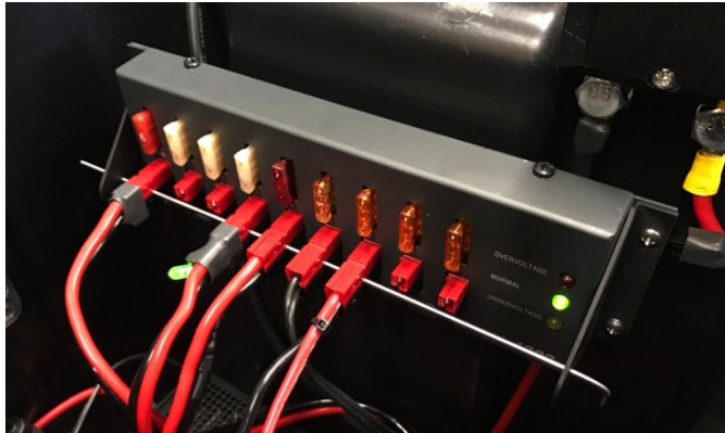
Figure 2.4.108. Fuse box for 12V power distribution
