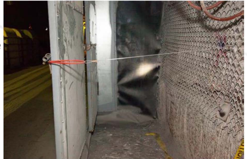
Air Lock Doors Wired Open
