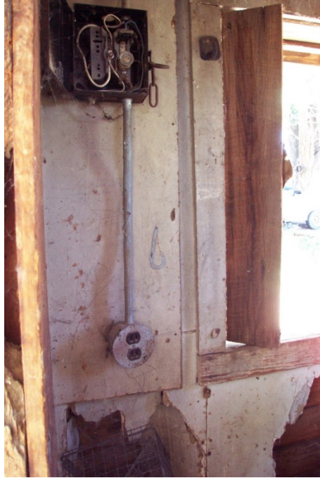
Figure 26. Interior of TA-20-20 with a single fuse electrical panel and a single electrical receptacle. Remnants of the original drywall interior with historic graffiti are still present.
