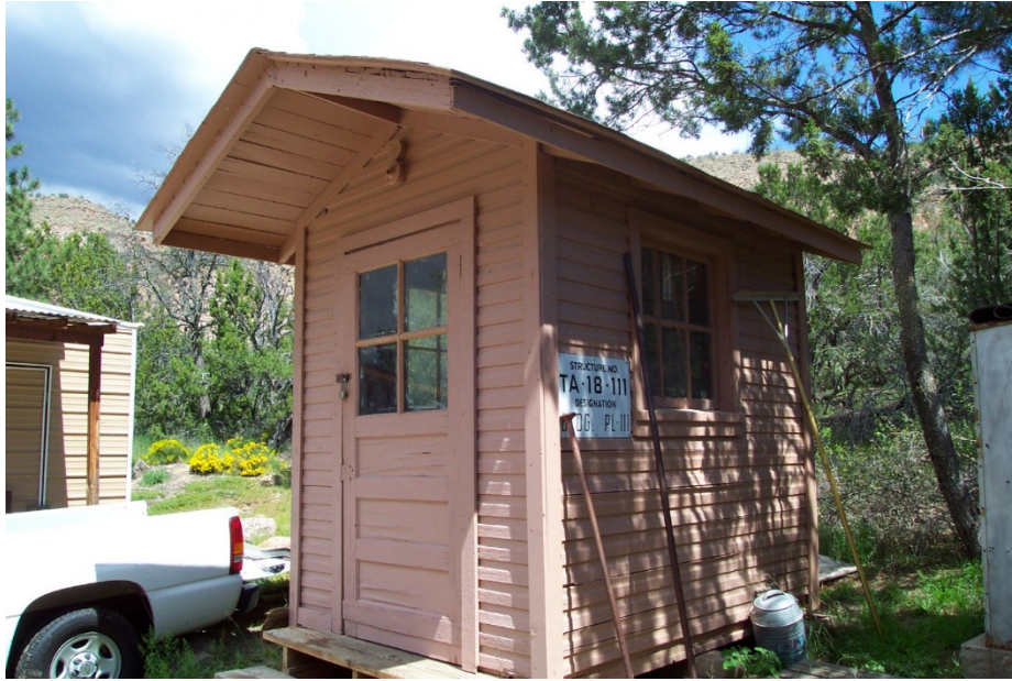
Figure 24. A portable Manhattan era guard station, TA-18-111, located in Bandelier National Monument. The building features a gable-style roof, rabbeted shiplap siding, and six-pane divided light windows.
