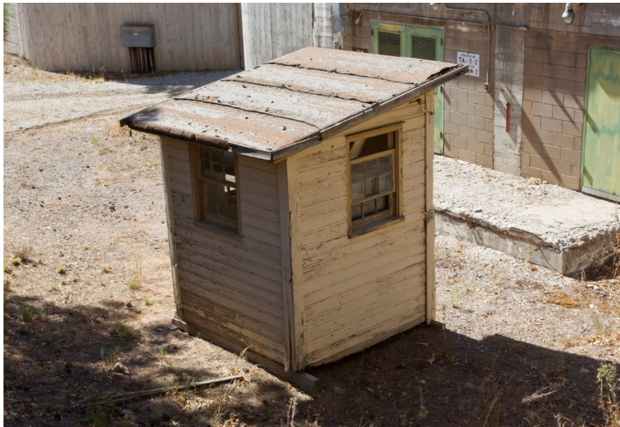
Figure 23. TA-8-172 as viewed from the left rear corner of the structure. Note the shed-style roof, roll roofing material, siding material, and six-over-six divided light, double hung windows.
