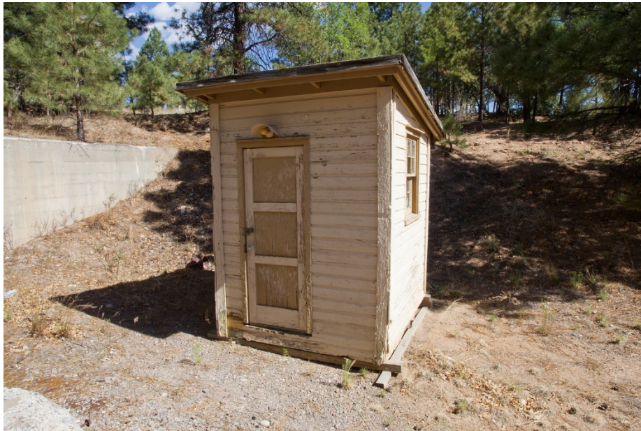
Figure 31. Exterior of TA-8-172, as viewed from the front, with custom sheet metal light fixture above the door. The three-panel door is likely not an original component.
