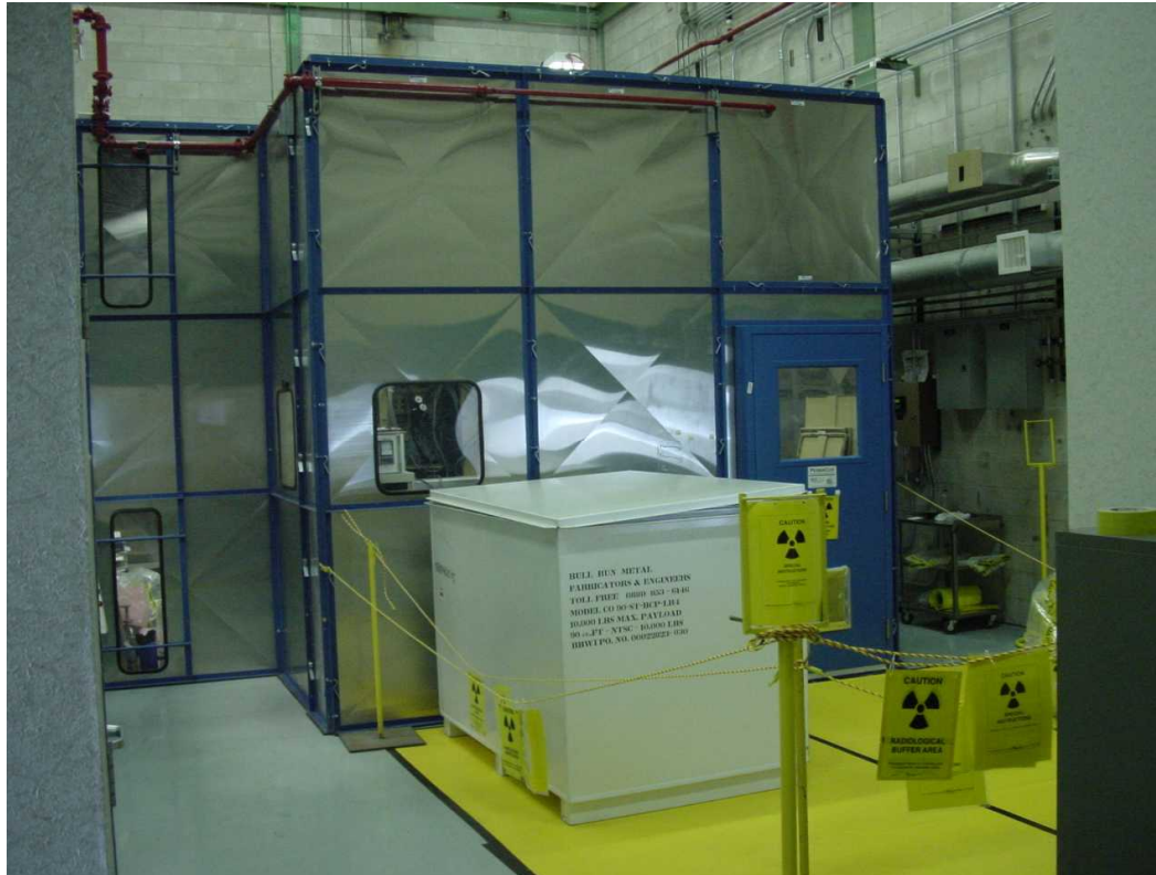
PermaCon enclosure housing TPE and ancillary equipment.
