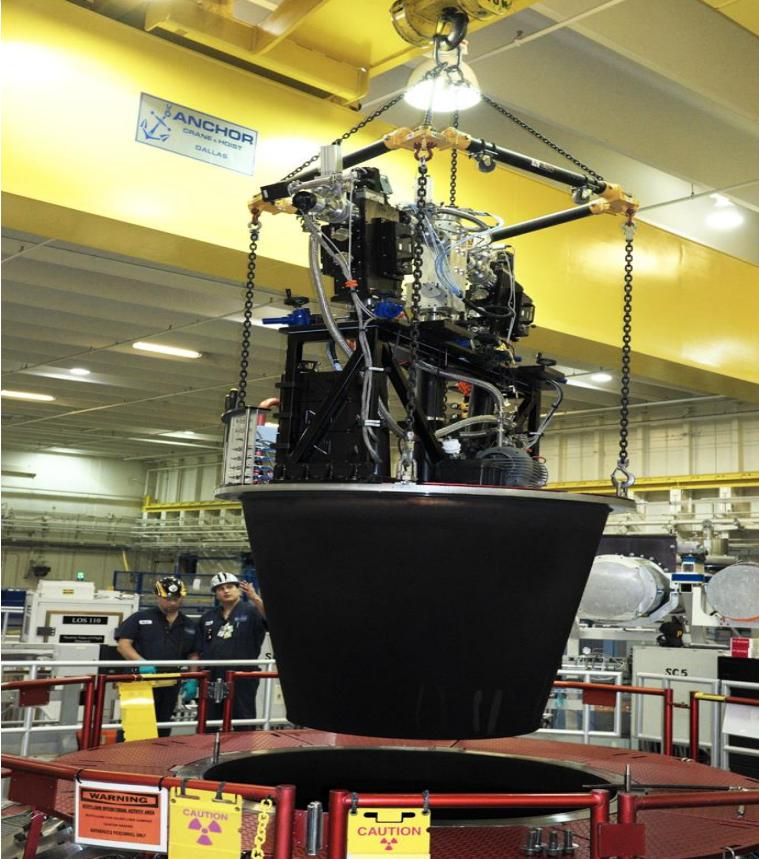
The array of opacity spectrometers is lowered into place with a 20 ton crane
