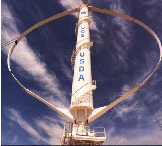
Figure 38. The Sandia 34 meter VAWT Testbed.
