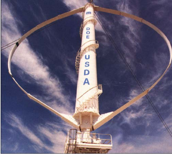
Figure 8. The Sandia 34 meter VAWT Testbed.
