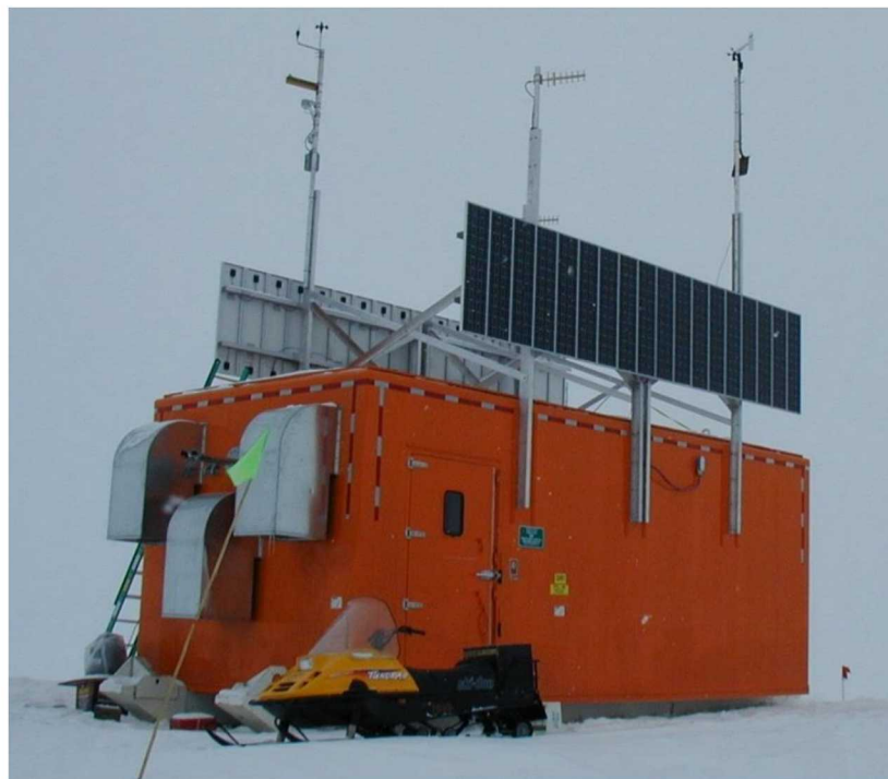
Figure 2.9.1 I55US Hybrid Power System (BOB)
