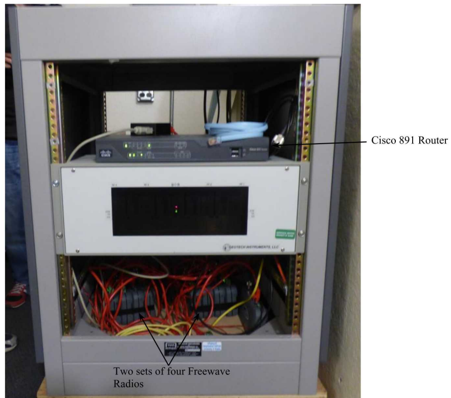
Figure 6.1.5 I55US Relay Radios
