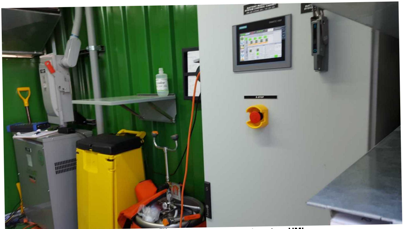
Figure 3 - Uni.System™ battery management system HMI
