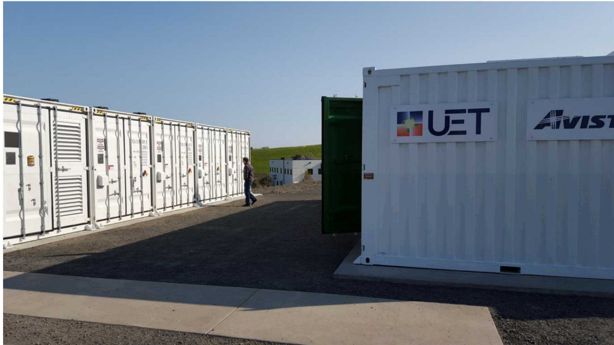
Figure 1 - 1 MW / 3.2 MWh UET Uni.System™ at Pullman, Washington
