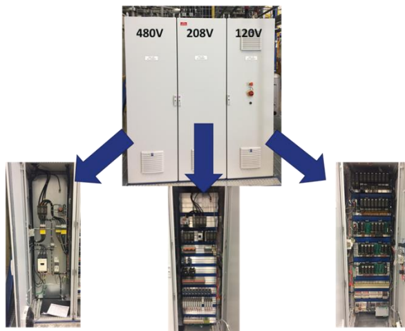
Figure 26: Mechanical, Electrical and Controls Installation
