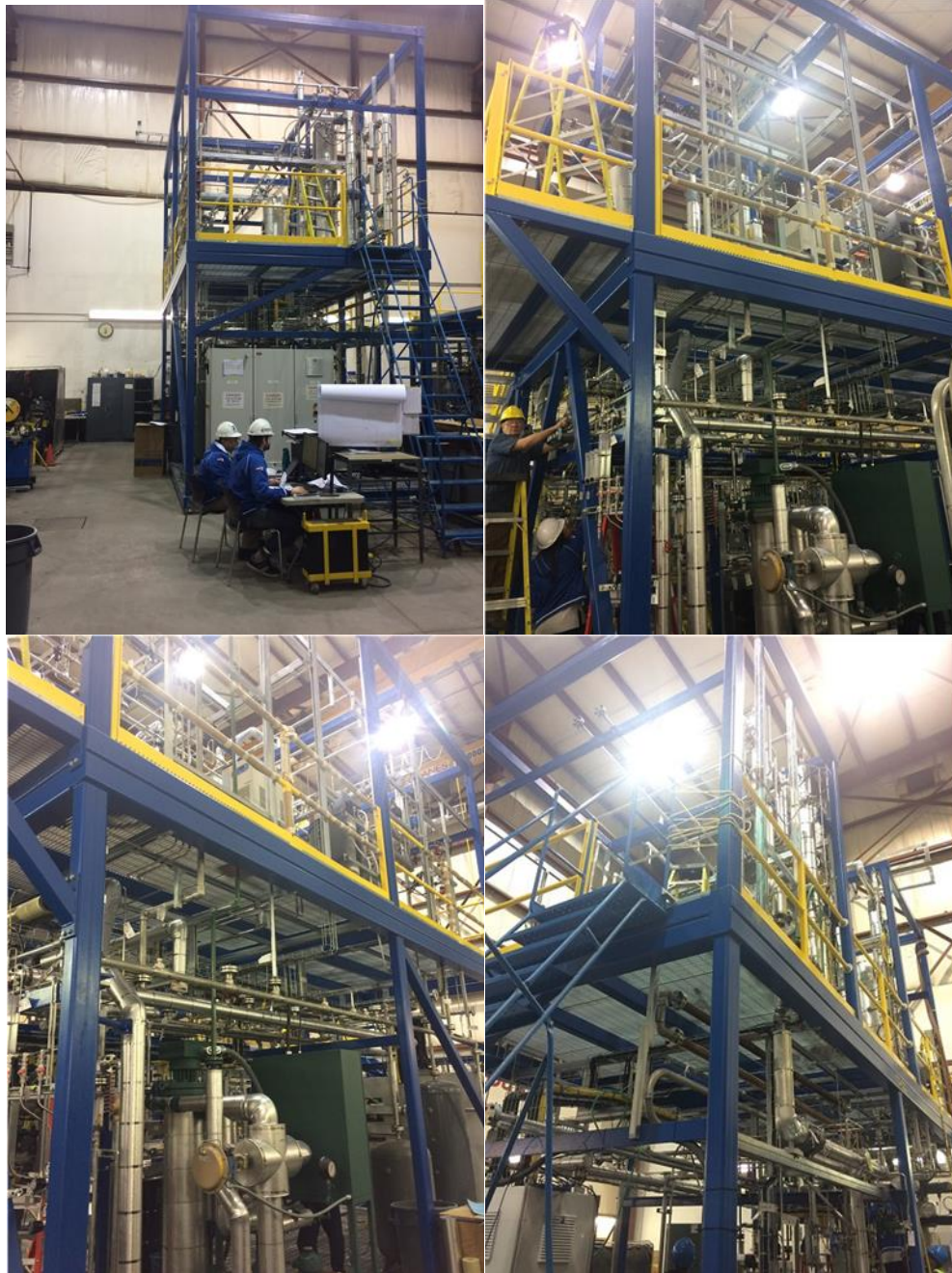
Figure 25: FAT Site Photos
