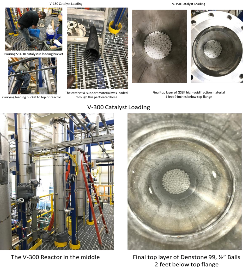
Figure 27: Photos of WGS and Sulphur Polishing Bed Catalyst Loading
