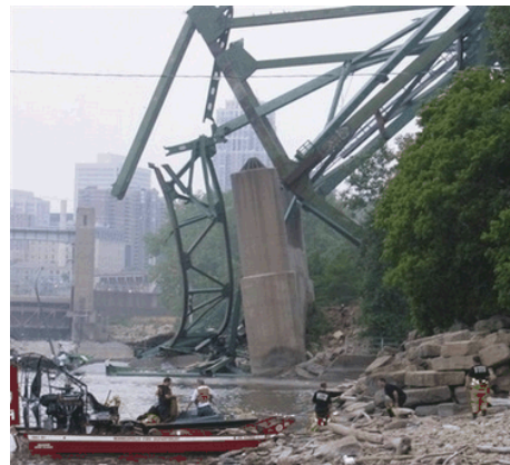
Minnesota I-35W Bridge Collapse
