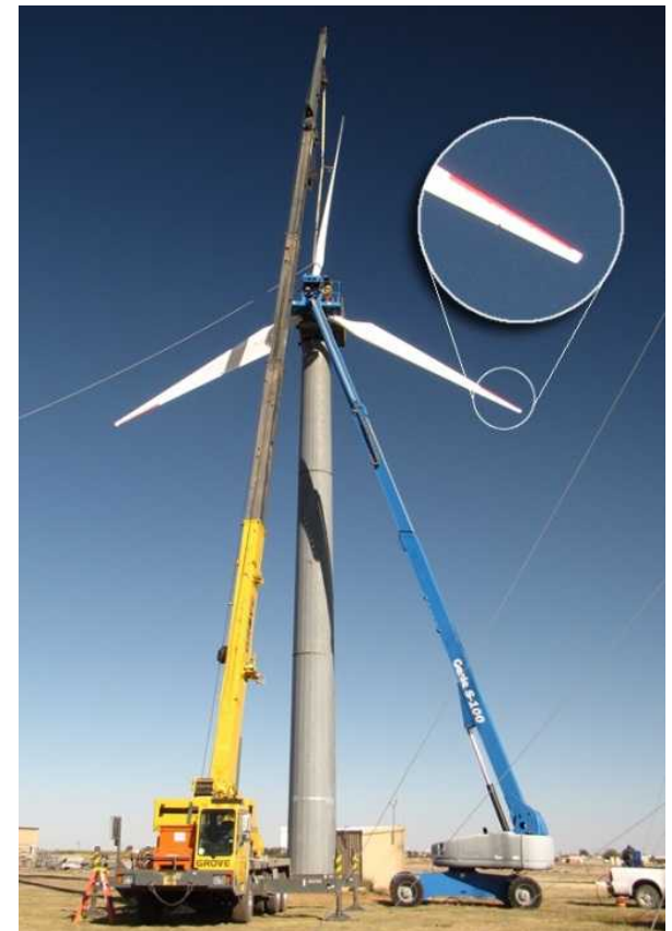
Rotors Installed on Wind Turbine
